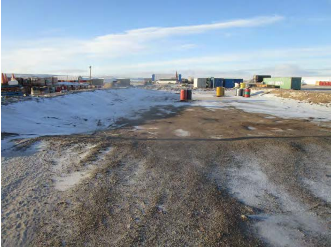
8. Barrel Fuel Containment. (MS-HWB-03)
