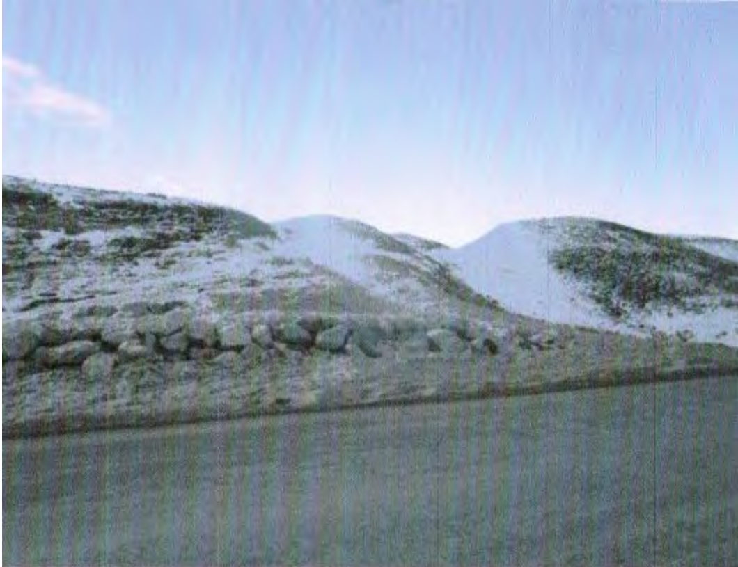
37. Armor Stone Used in Road Cut Area km 91
