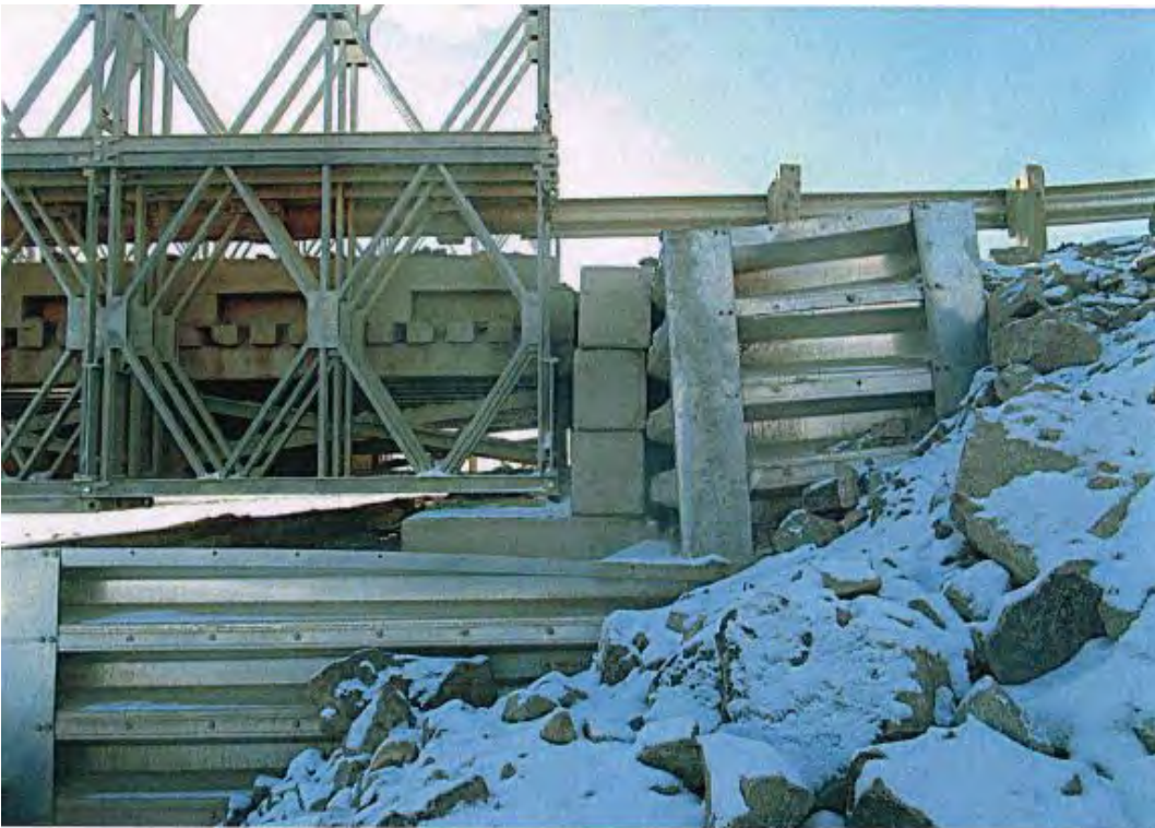
33. Bridge Abutment @ km 63 (Note Space)
