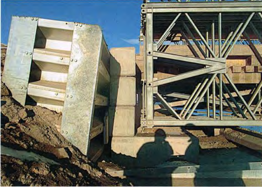
34. Bridge Abutment @ km 80 (Note Space)
