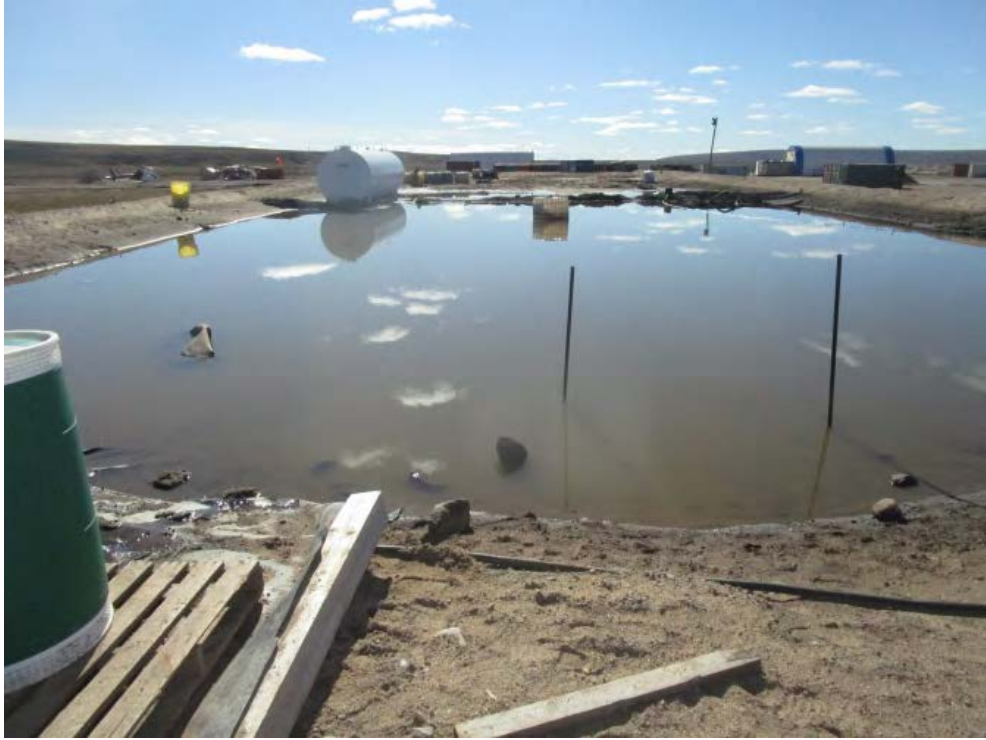
1. Bulk Fuel Storage Facility (MS-HWB-7)
