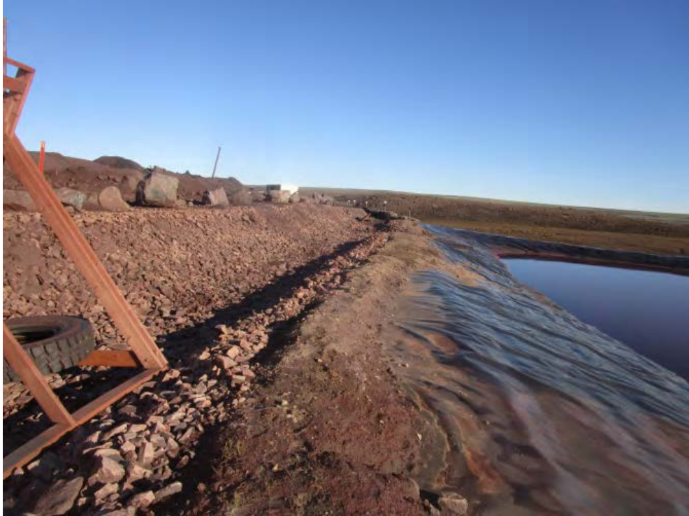
17. Crusher Pad Drainage Containment
