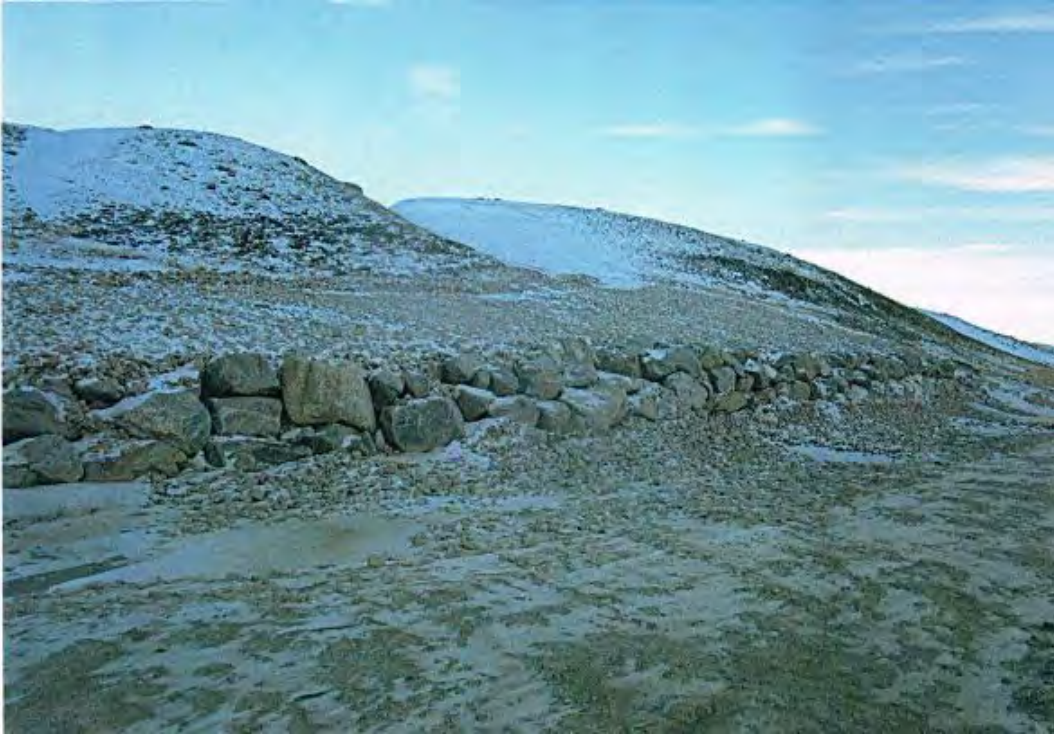
38. Armor Stone Used in Road Cut Area km 91
