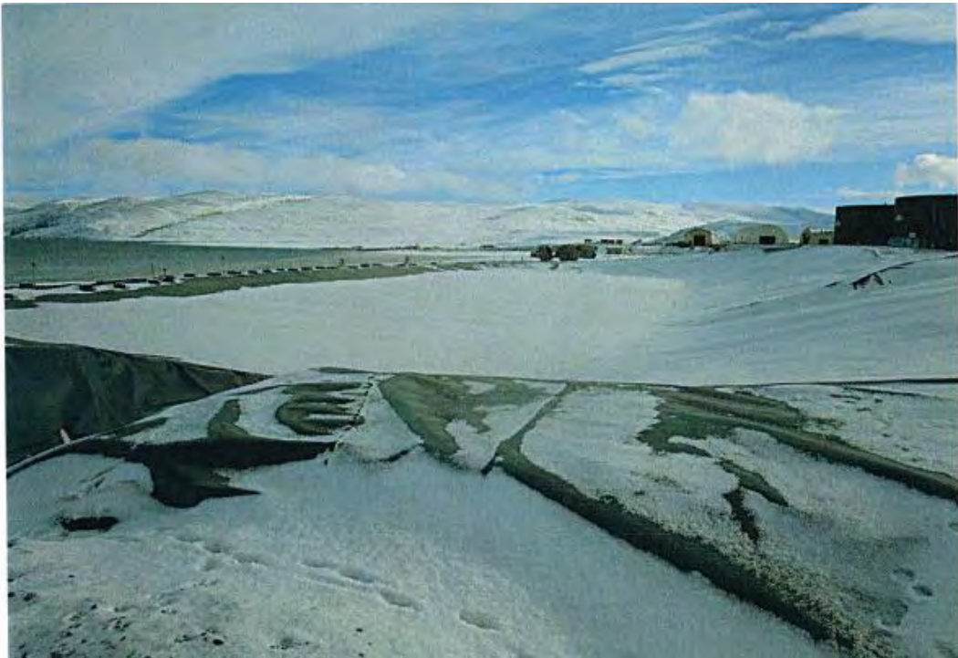
30. Milne Port Ore Stockpile Sedimentation Pond East (MP-05)
