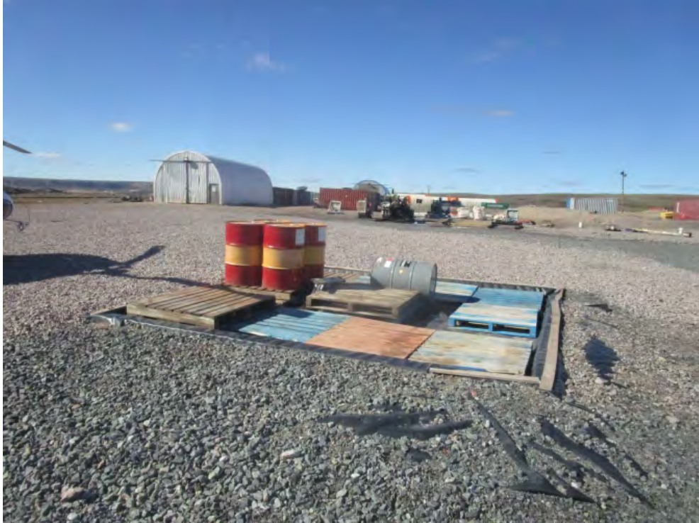
7. Temporary Helicopter Fuel Containment
