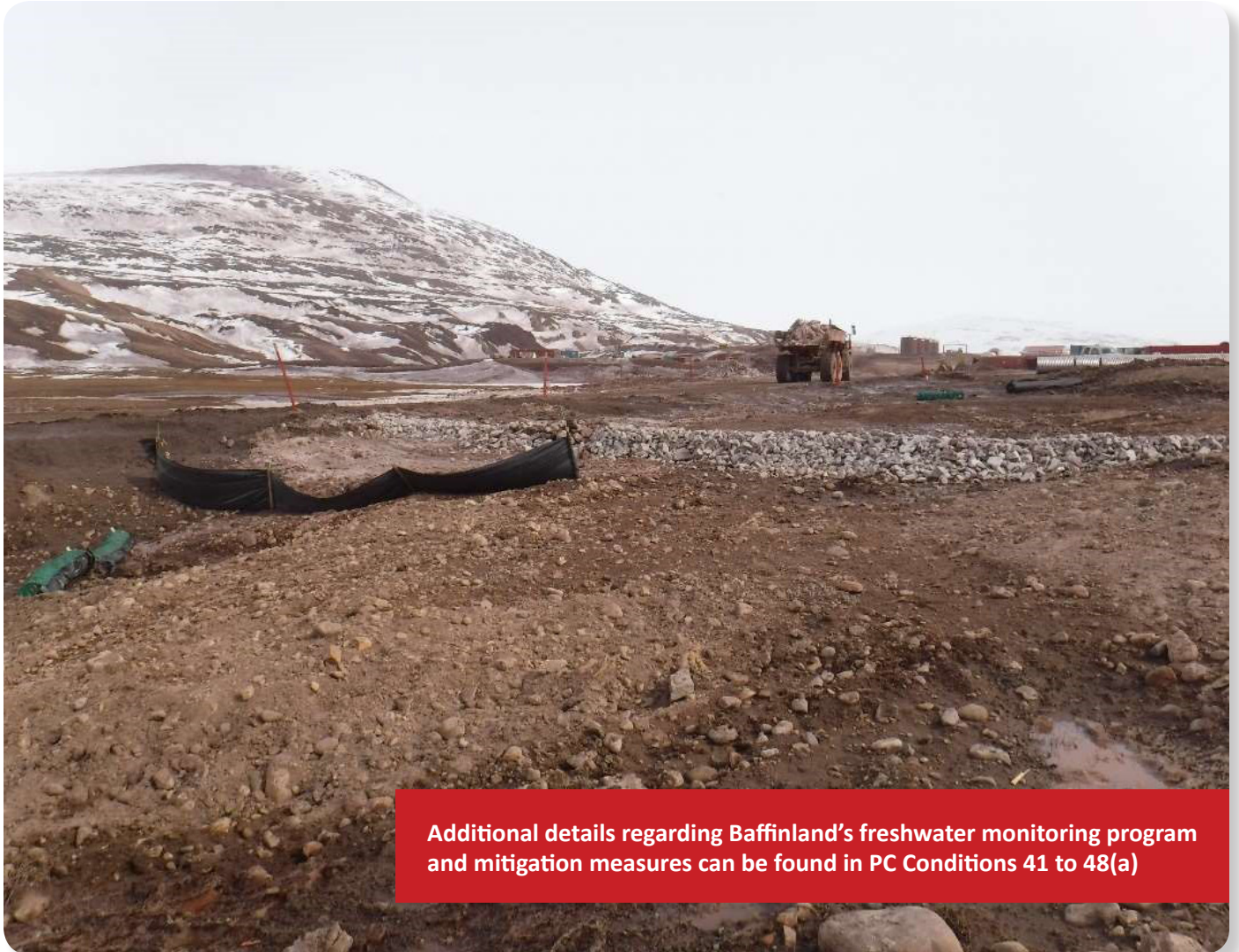
May 16, 2017 - Construction of check dam north of culvert CV-186 (Sheardown Lake Tributary)
