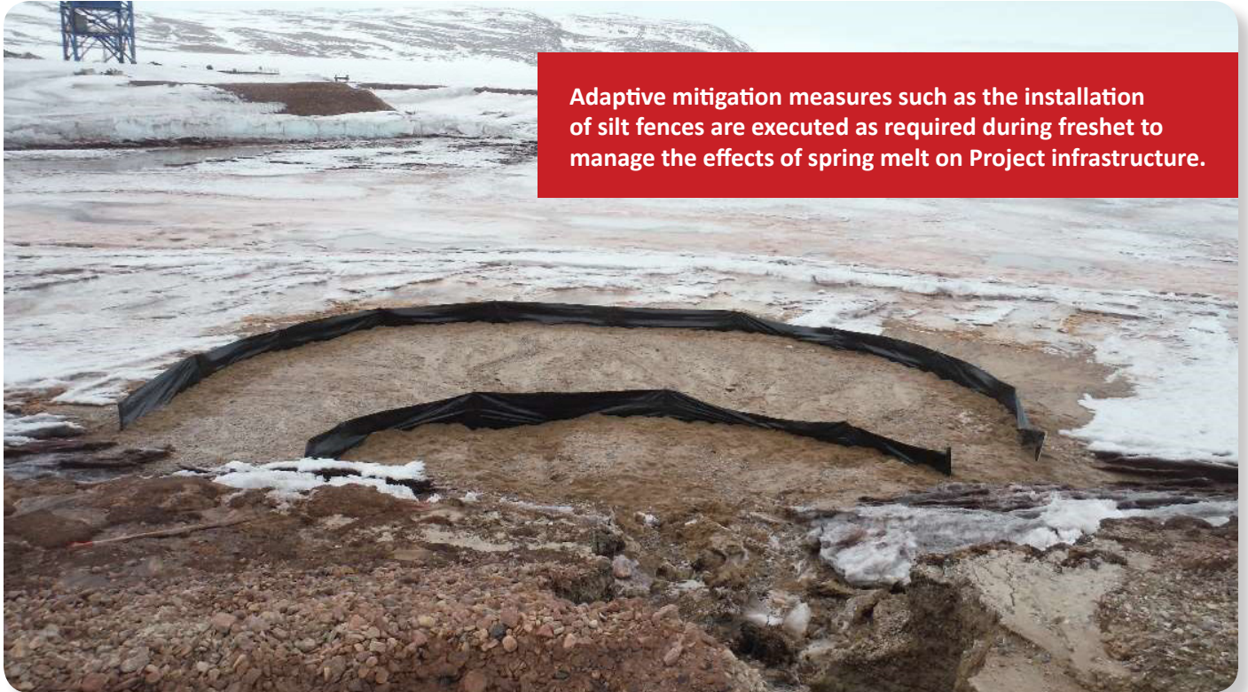
May 26, 2017 – Silt fences installed to contain sediment released as a result of Milne Port East Sedimentation Pond (MP-05) overflow on May 25, 2017
