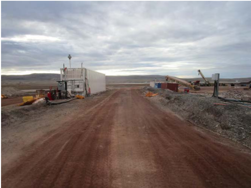
32. Fuelling Facility (OHT Laydown)
