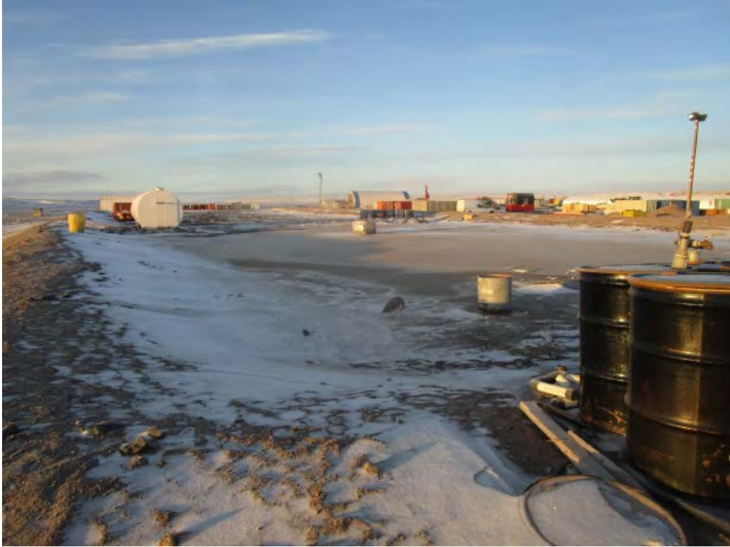
1. Bulk Fuel Storage Facility. (MS-HWB-7)
