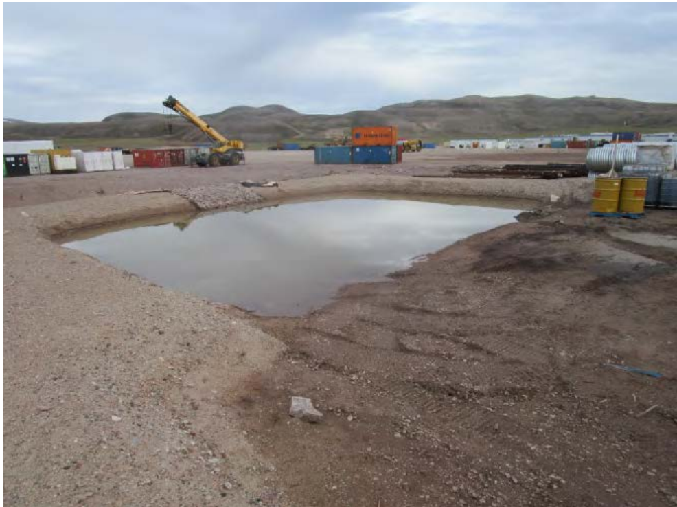
2. Generator Fuel Containment
