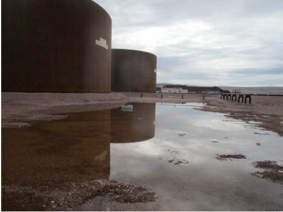
23. Fuel Tank Farm
