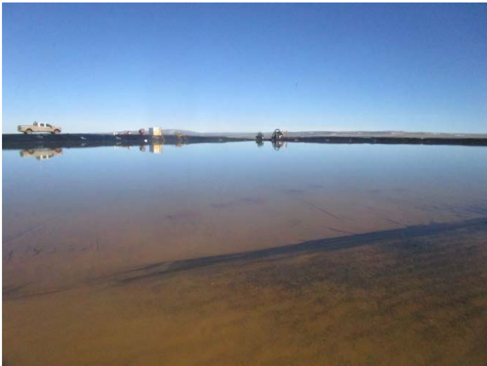
18. Waste Pile Drainage Containment
