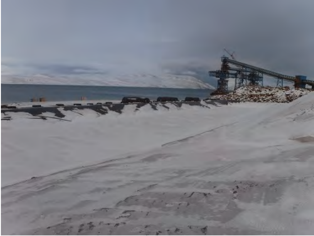
31. Milne Port Ore Stockpile Sedimentation Pond West (MP-06)
