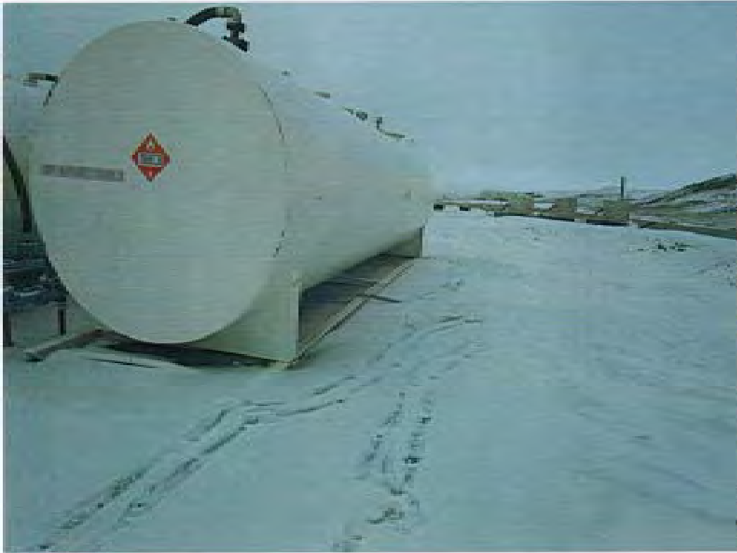
19. Jet 'A' Fuel Containment.
