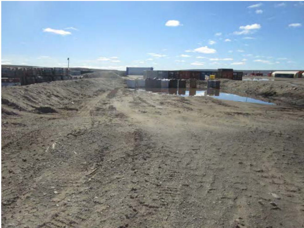
8. Barrel Fuel Containment MS-HWB-4
