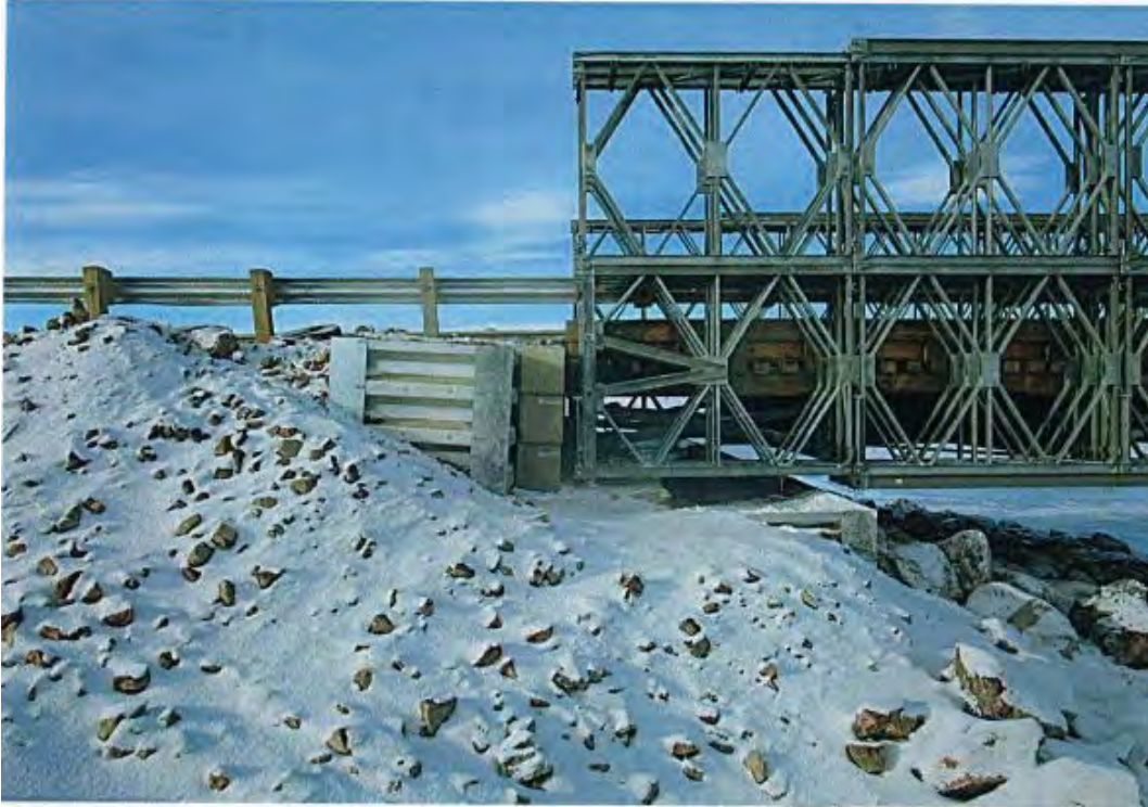
32. Bridge Abutment @ km 97 (Note Space)
