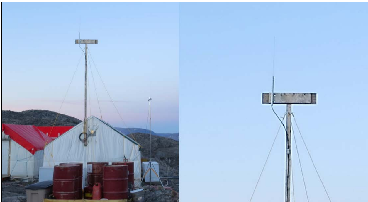
FIGURE 8. Antenna for the Automatic Identification System (AIS) was mounted on a wooden mast attached to the kitchen tent at the Bruce Head camp.
