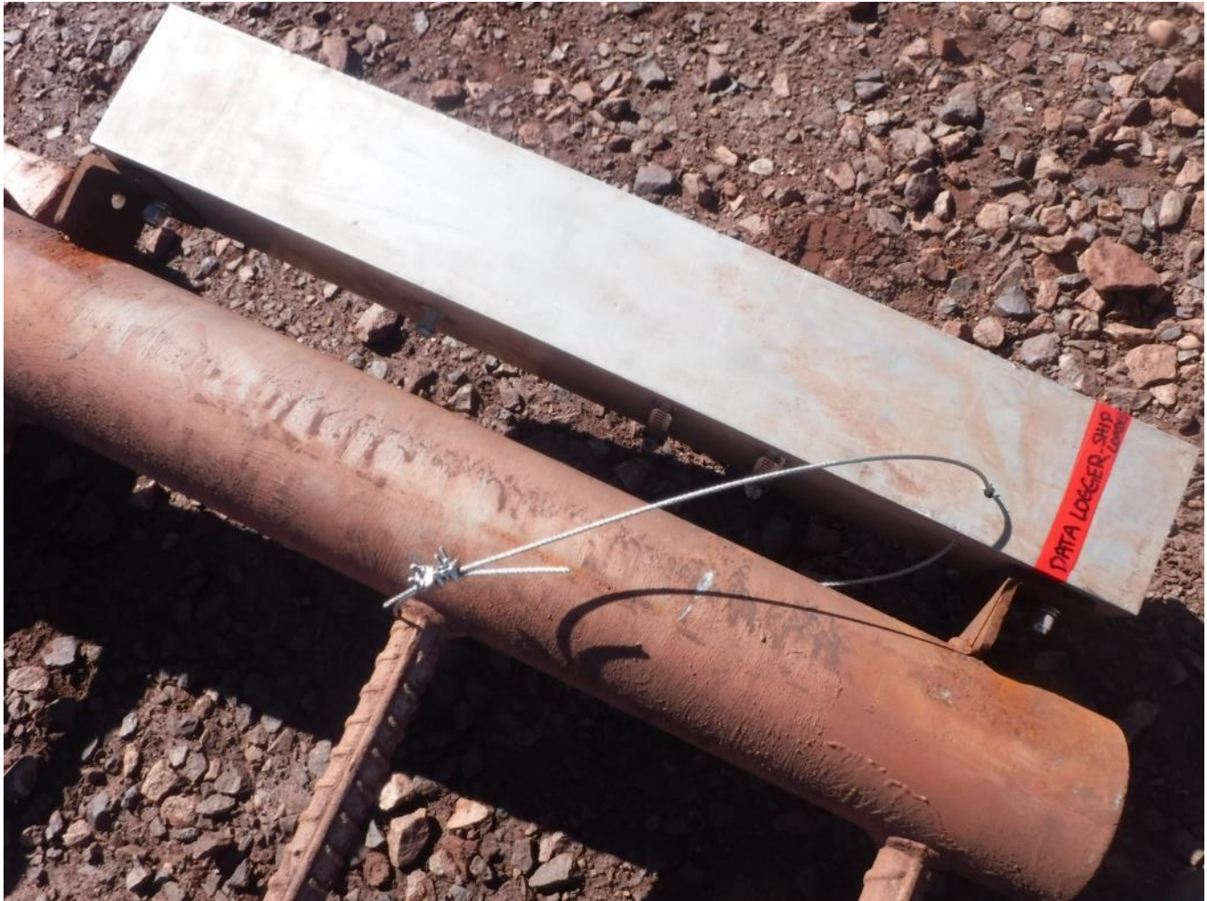
Figure 2: Hardware attaching aluminum tube to steel L brackets and wire rope for redundancy of the L bracket attachments.
