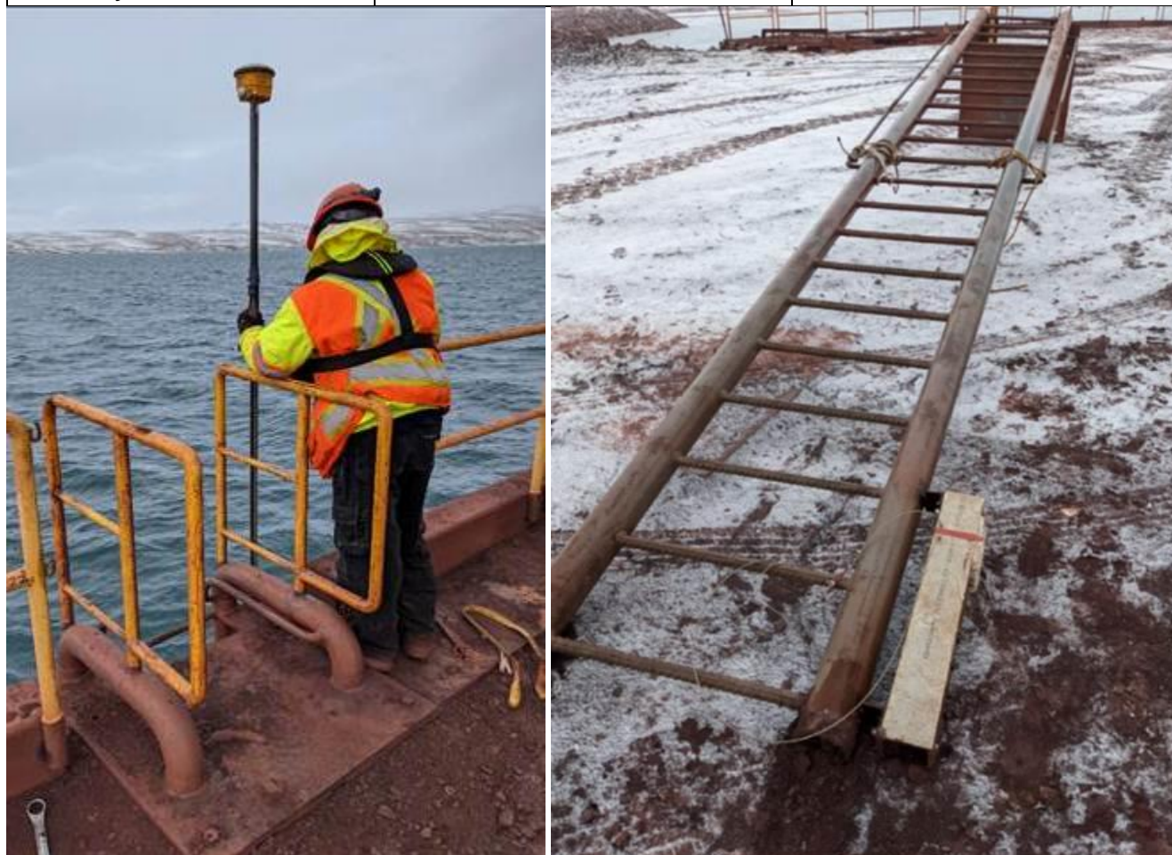
Figure 1: Left: RTK Survey of the ore dock ladder top plate. Right: Ore dock ladder following removal, with the tide gauge housing shown on the bottom right of the ladder. (Ritgen, 2020)
