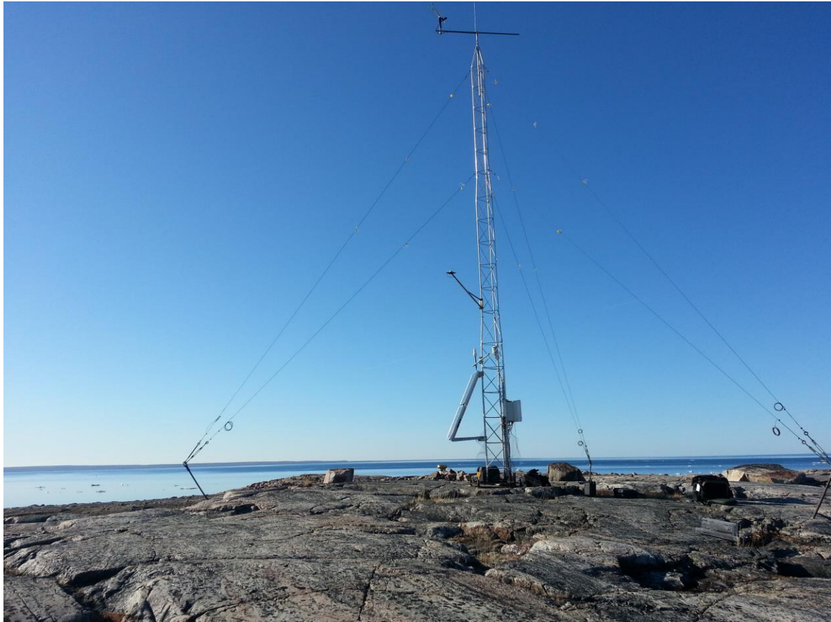
Figure 8: Steensby met station (picture taken during 2014 trip - looking towards the West)
