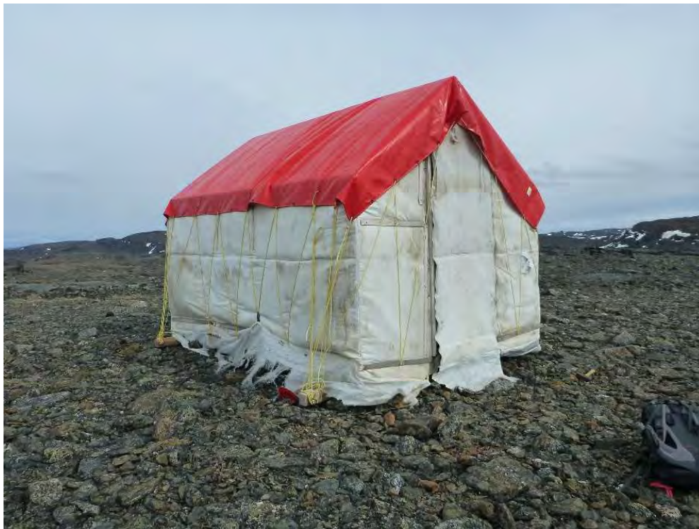
PHOTO 9 – Eqe Bay Survival Shack Structure
