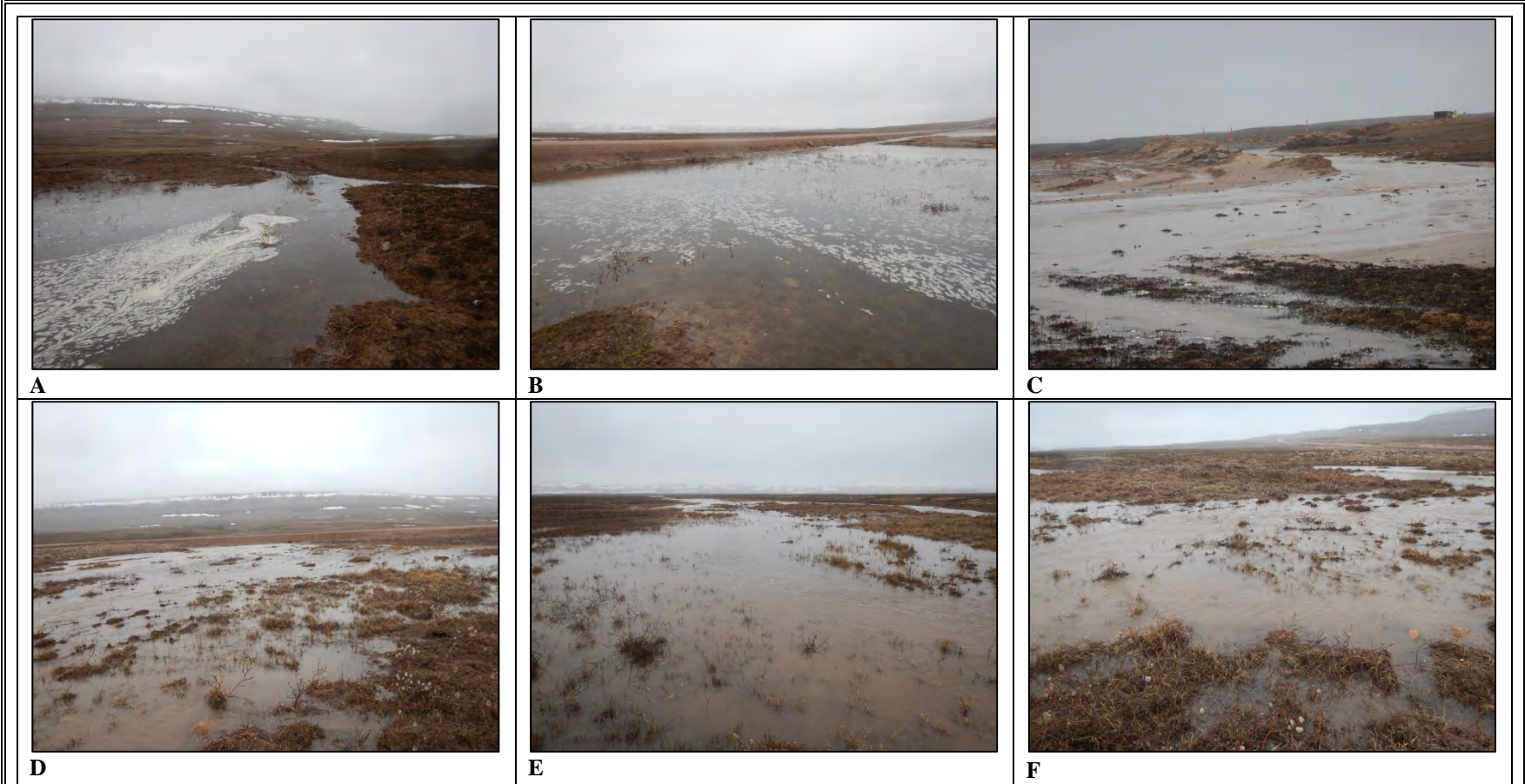
Photos 1. Photographs upstream (top) and downstream (bottom) of the Tote Road crossing CV-030: (A,D) looking upstream; (B,E) looking downstream; (C) diversion flow from CV-031; and (F) looking across flooded terrestrial vegetation downstream.
