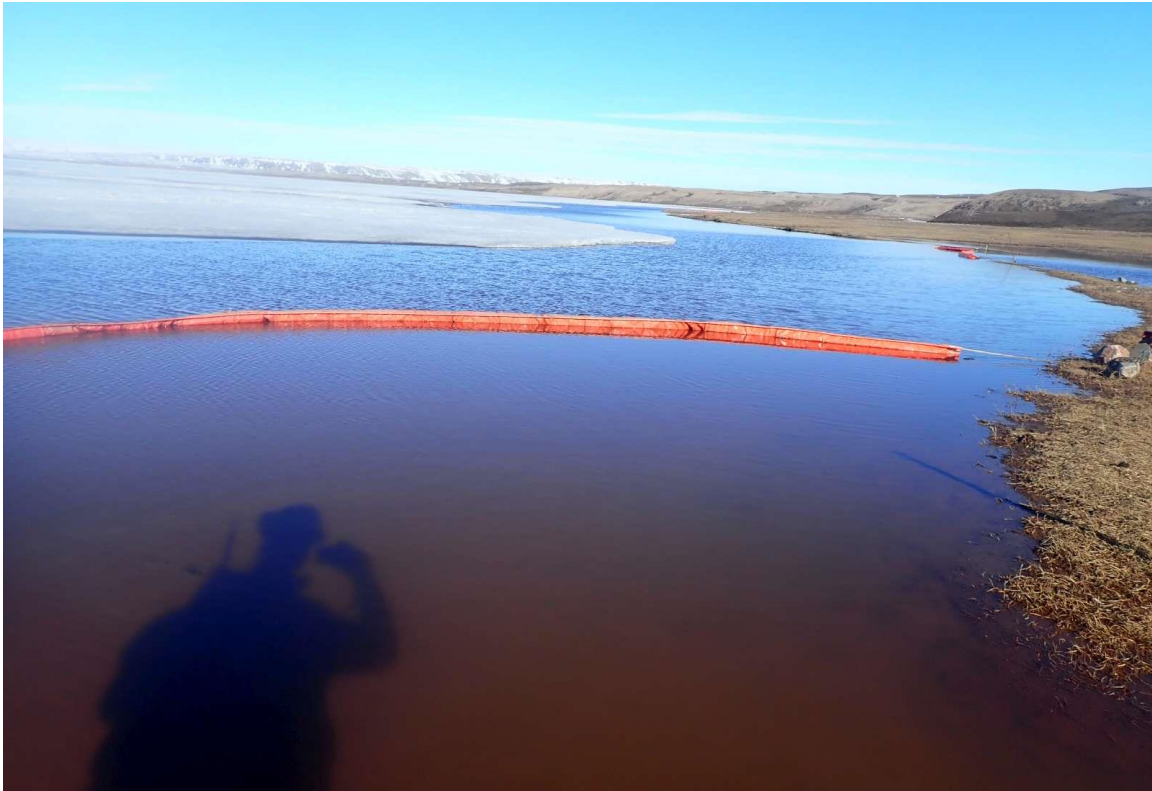
Photo 9: CLSP Outfall into Silt Curtain on June 11, 2020
