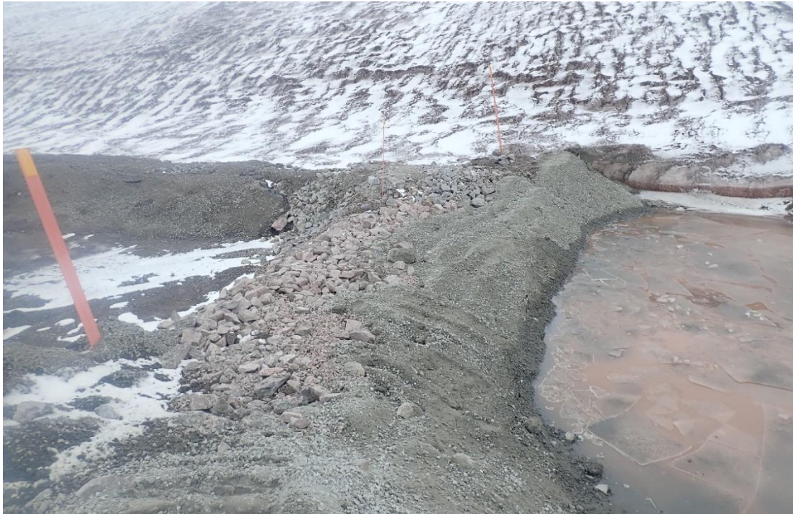
Photo 7: Camp Lake Check Dam Improvements on May 21, 2020
