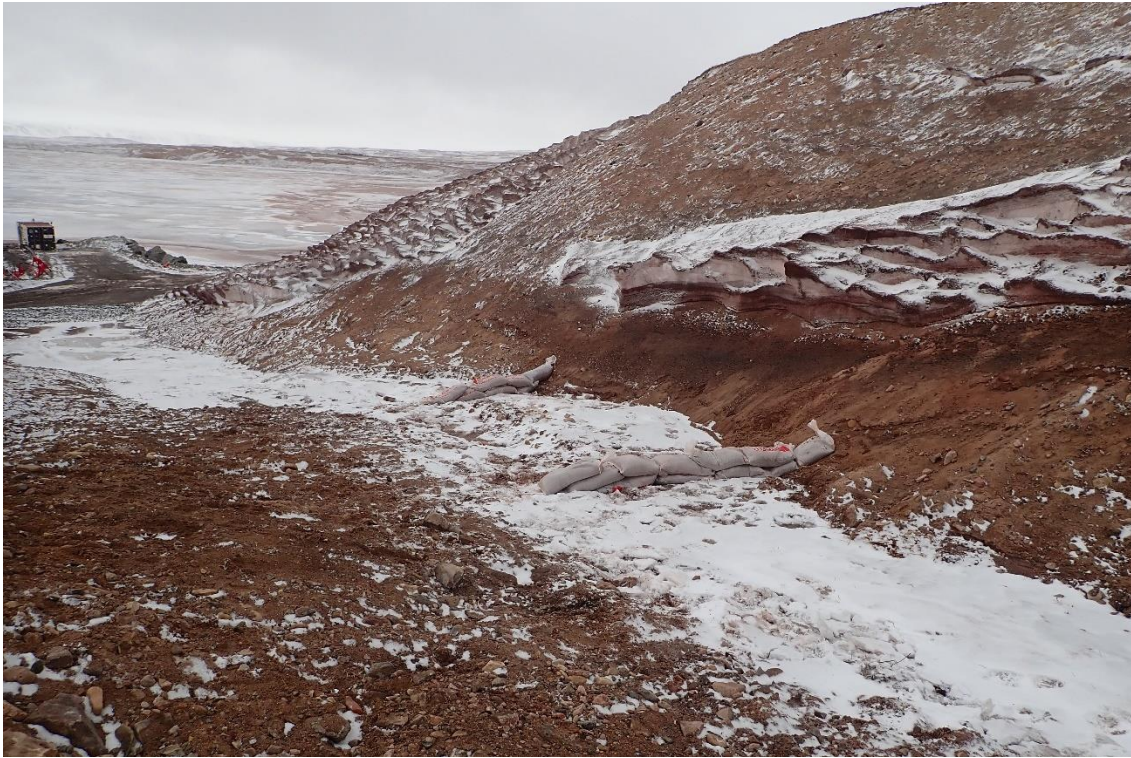
Photo 5: Camp Lake Check Dams with Sand Bags on May 18, 2020
