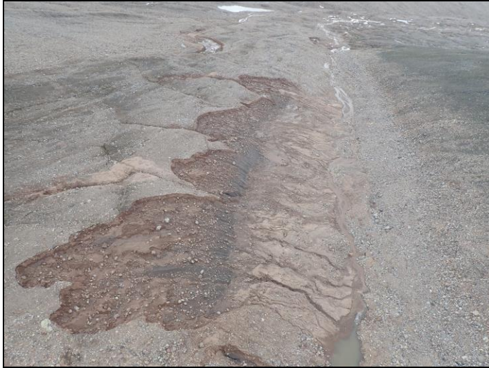
Figure 4. Aerial photograph of sloughed hillside.
