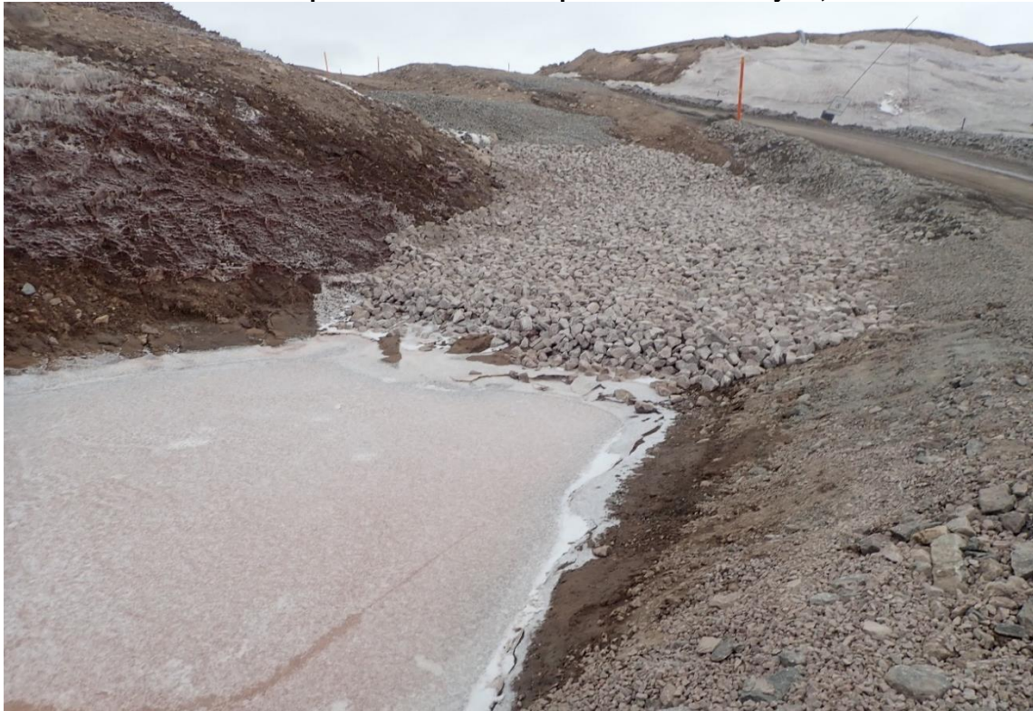
Photo 8: Camp Lake Slope Rip Rapping on May 23, 2020
