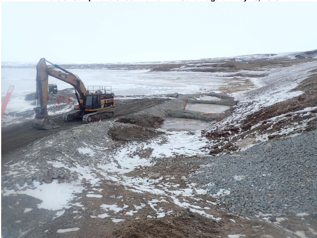
Photo 6: Camp Lake Settling Improvements on May 21, 2020
