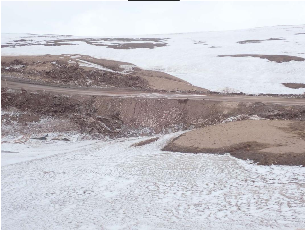
Photo 1. Snow Clearing at the Outlet of BG-01 (May 14, 2020)
