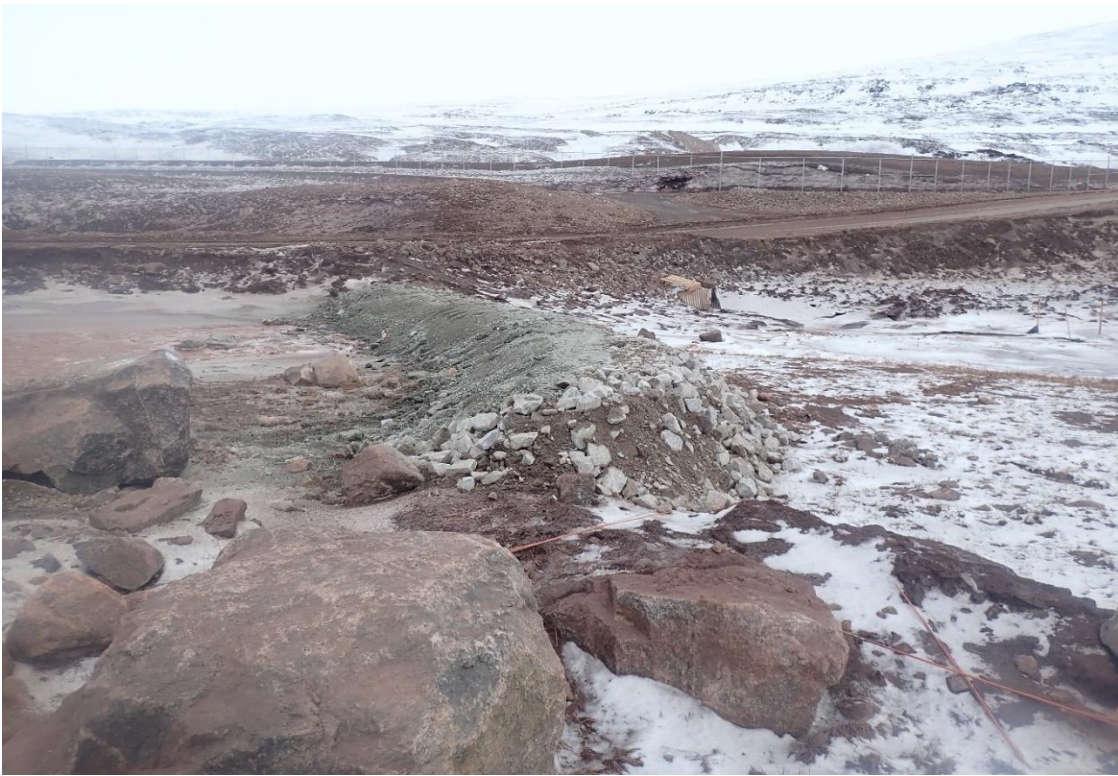
Photo 5. Check Dam Reinforcement and Expansion at the Inlet of CV-187 (May 20, 2020)
