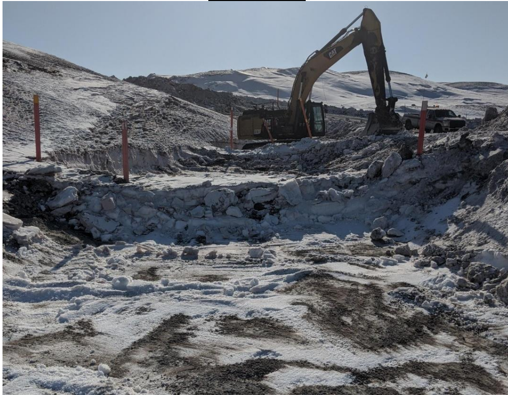
Photo 1. Snow Removal at the Camp Lake Check Dams on April 21, 2020
