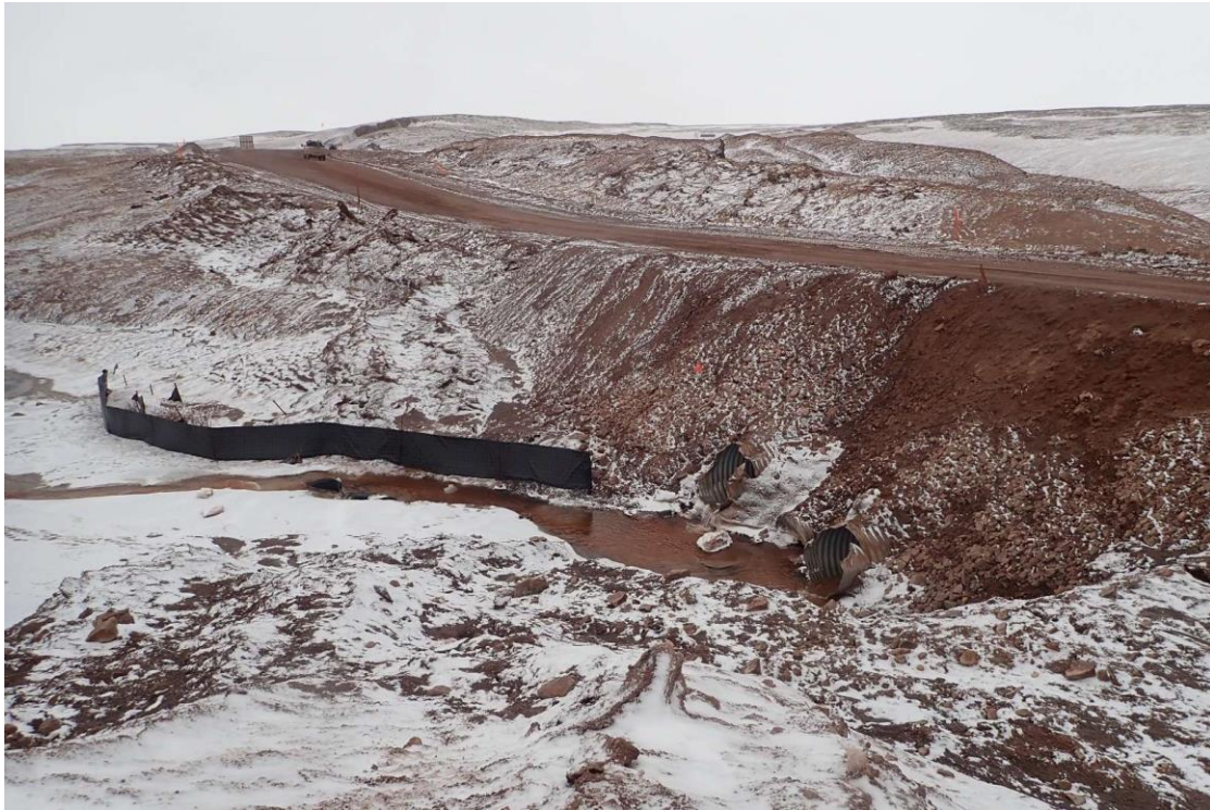
Photo 5. Silt Fencing at the Outlet of BG-01 (May 18, 2020)
