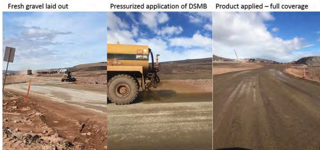
Photo 3-2 Dust Stop® application to the Tote Road, 2019.
