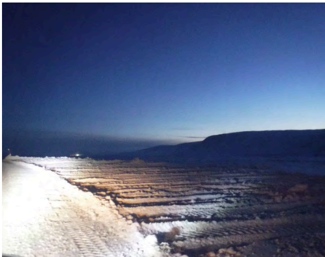
Photo 5-7 Example of snow bank management on side of Tote Road near km 15 to make sure they do not exceed the maximum snow bank height, December 25, 2018.
