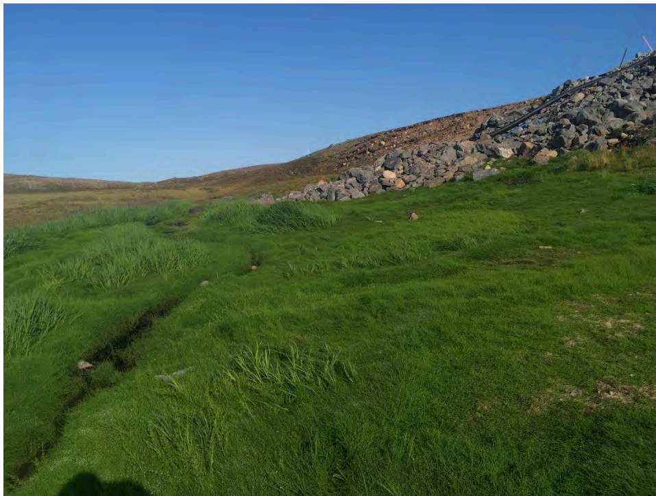
Photo 4-7 Overview of the sewage/effluent discharge area at the Mine Site looking upslope towards the outlet pipe and rock armor, 31 July 2019.
