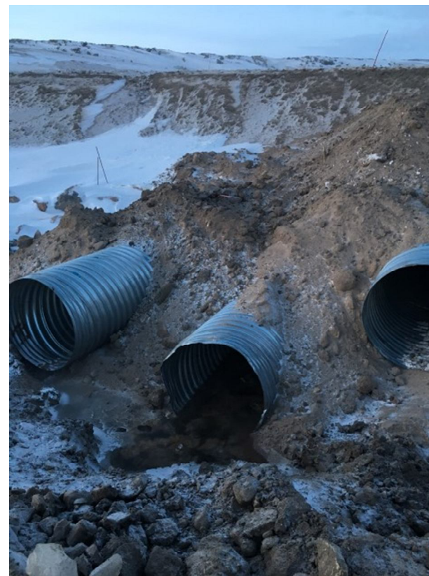
Figure 2. BG01 US mid-installation 17-10-05
