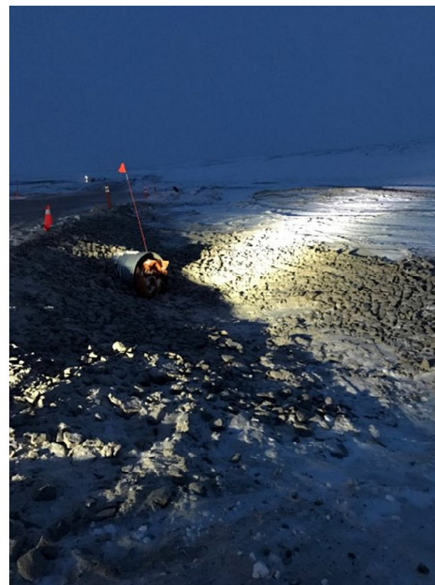
Figure 15. CV106 DS post-culvert extension 17-12-03
