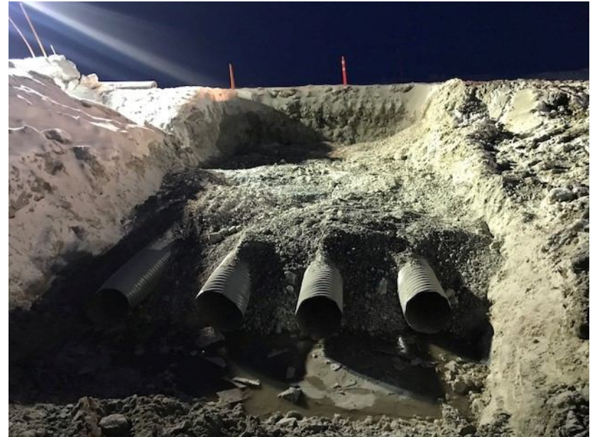
Figure 11. CV059 DS during culvert replacement 17-12-18
