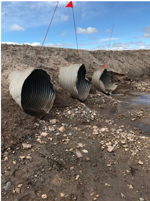
Figure 27. CV216 DS pre-culvert extension 17-07-24
