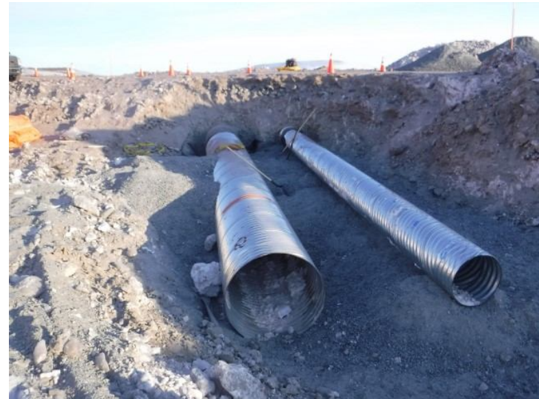
Figure 24. CV187 DS culvert extension 17-04-20
