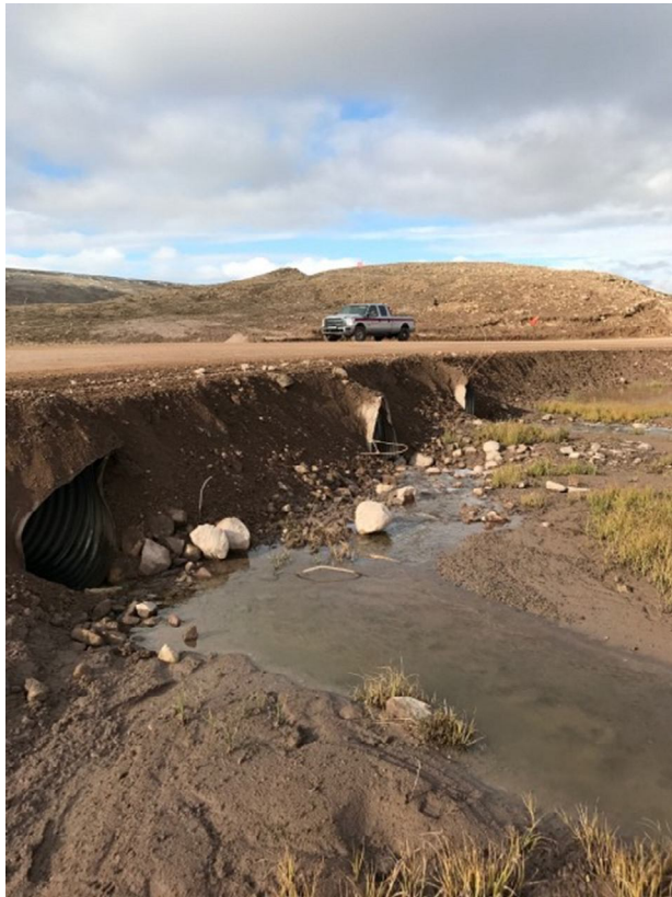
Figure 16. CV112 DS pre-culvert extension 17-09-11
