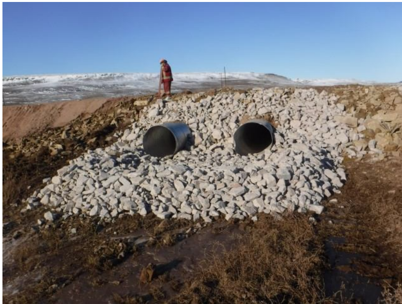
Figure 9. BG 32 DS culvert extension completed 17-09-23
