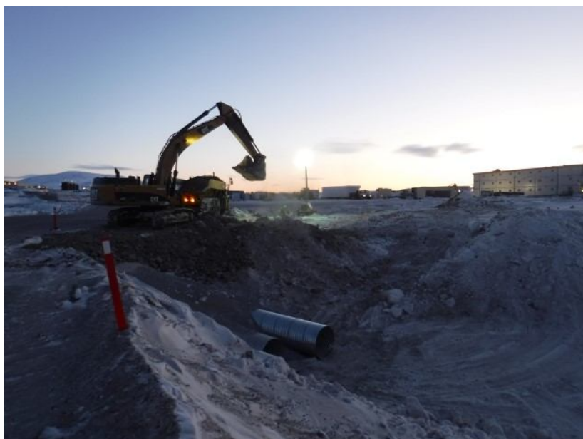
Figure 21. CV186 DS culvert installation 17-11-27
