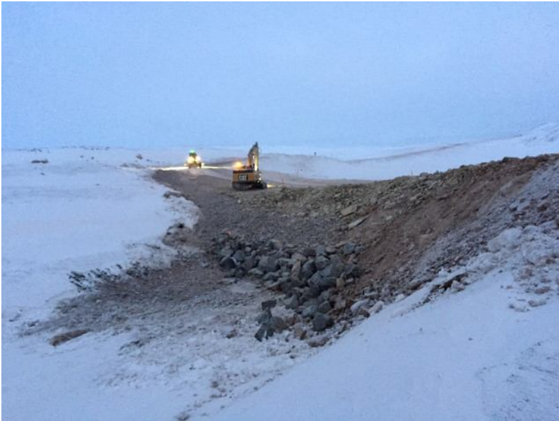
Figure 6. BG29 DS culvert extension installed 17-11-09
