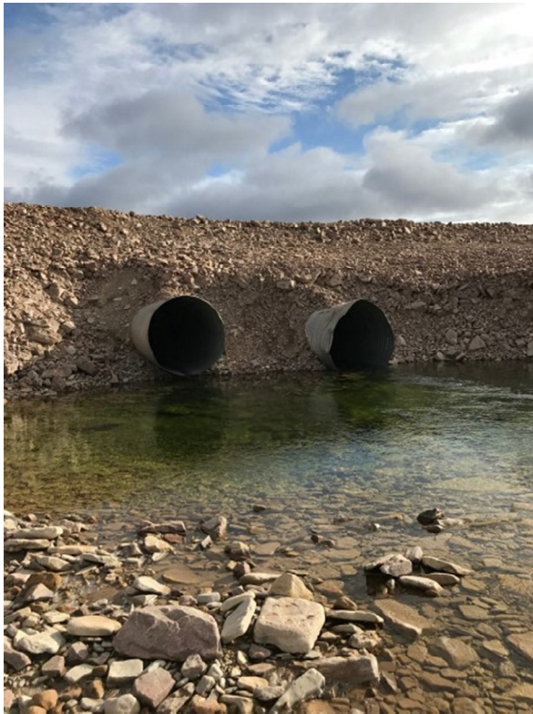
Figure 12. CV099 DS pre slope embankment reinforcement 17-09-11
