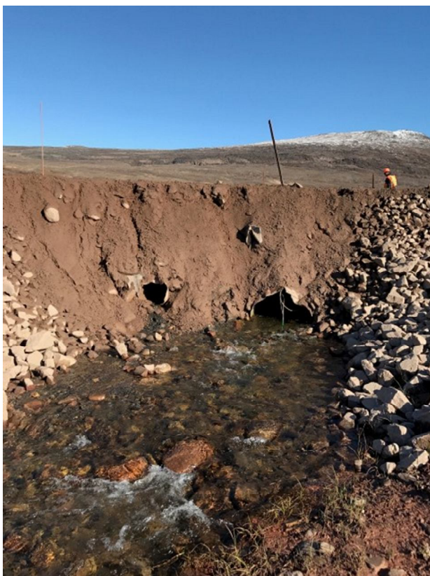
Figure 19. CV186 DS pre-culvert extension 17-09-02
