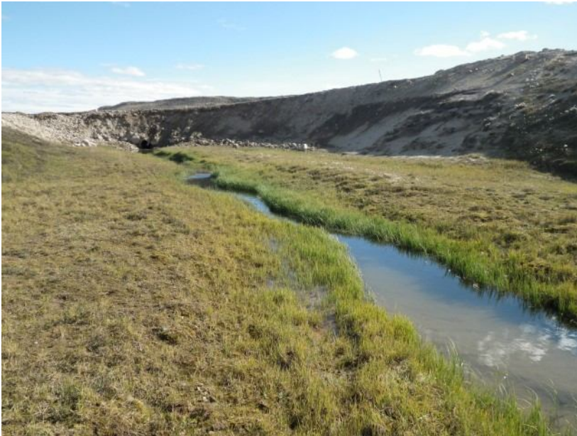
Figure 4. BG29 DS pre-culvert extension 16-08-12
