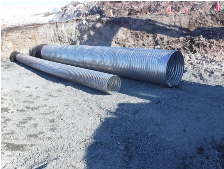
Figure 23. CV187 US culvert extension 17-04-23
