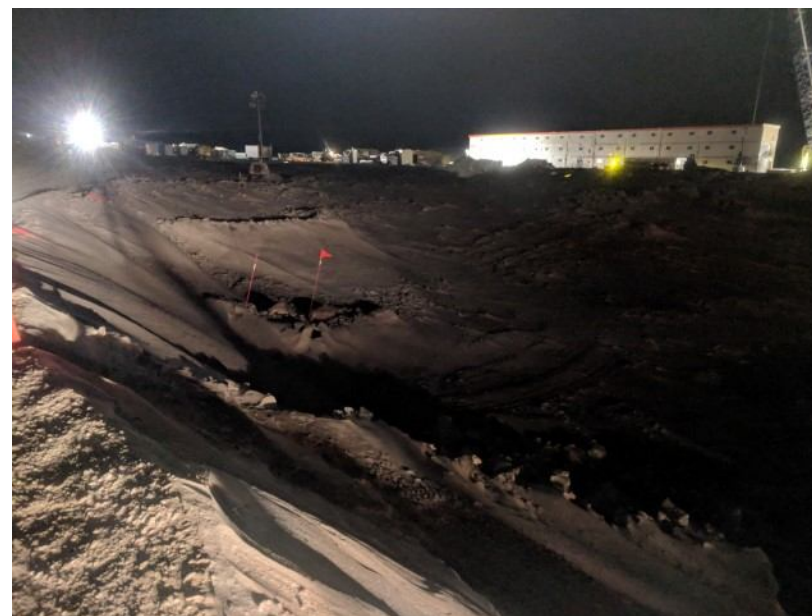
Figure 22. CV186 DS culvert extension completed 17-12-01
