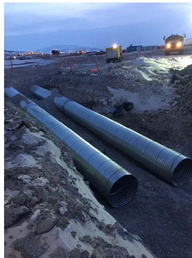
Figure 20. CV186 DS culvert extension 17-11-28
