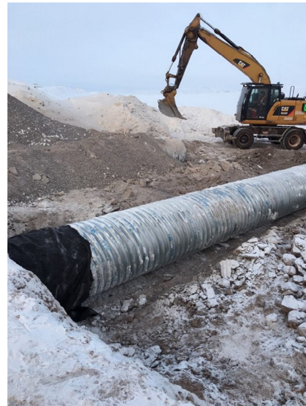
Figure 17. CV112 DS culvert extension installation 17-11-04
