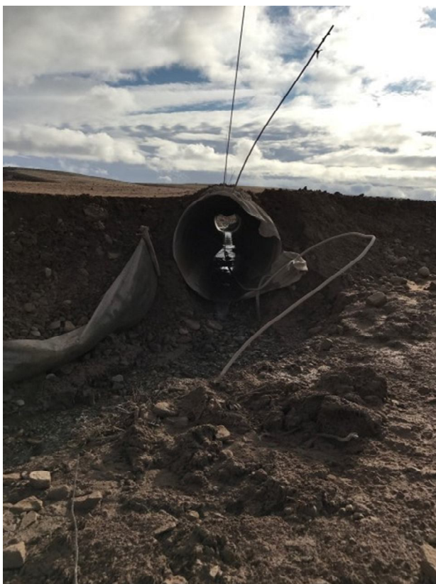
Figure 14. CV106 DS pre-culvert extension 17-09-11
