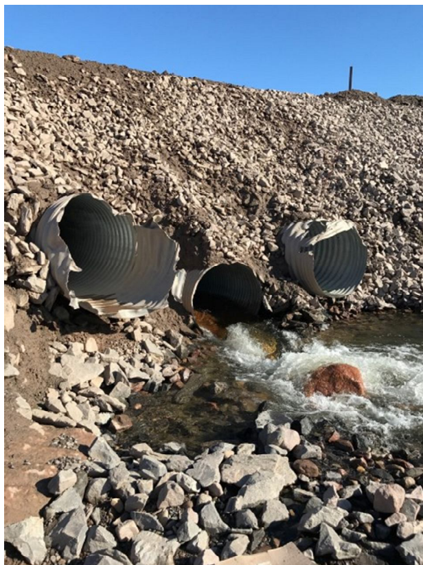
Figure 1. BG01 DS pre-construction 17-09-02
