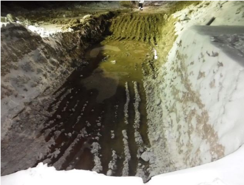
Figure 10. CV059 DS after historical culvert removal 17-12-09
