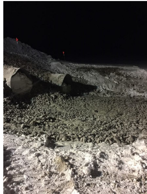
Figure 13. CV099 DS post slope embankment reinforcement 17-12-03
