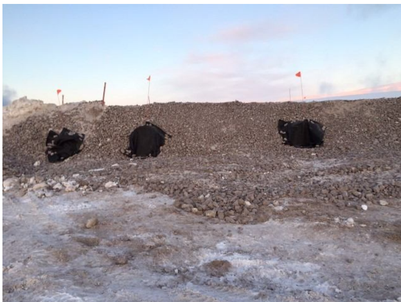
Figure 18. CV112 DS post-culvert extension 17-11-04
