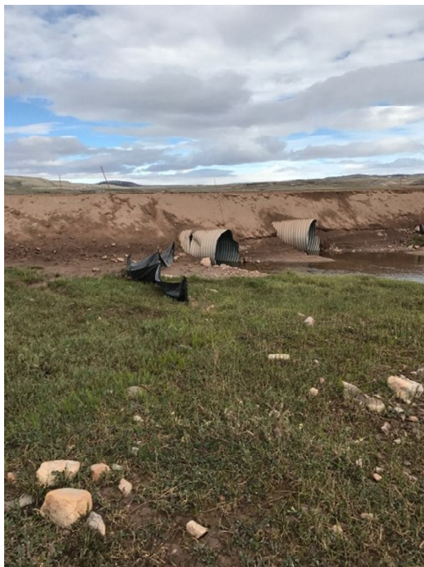
Figure 7. BG32 DS pre-culvert extension 17-07-24
