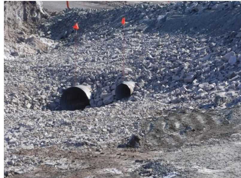
Figure 26. CV187 DS culvert extension completed 17-04-24
