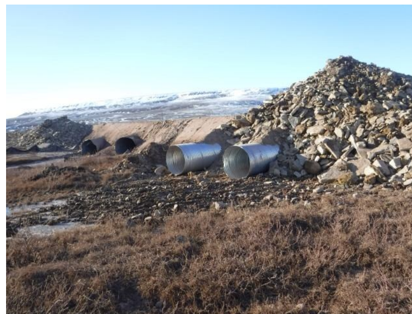
Figure 8. BG32 DS mid-culvert extension installation 17-09-22
