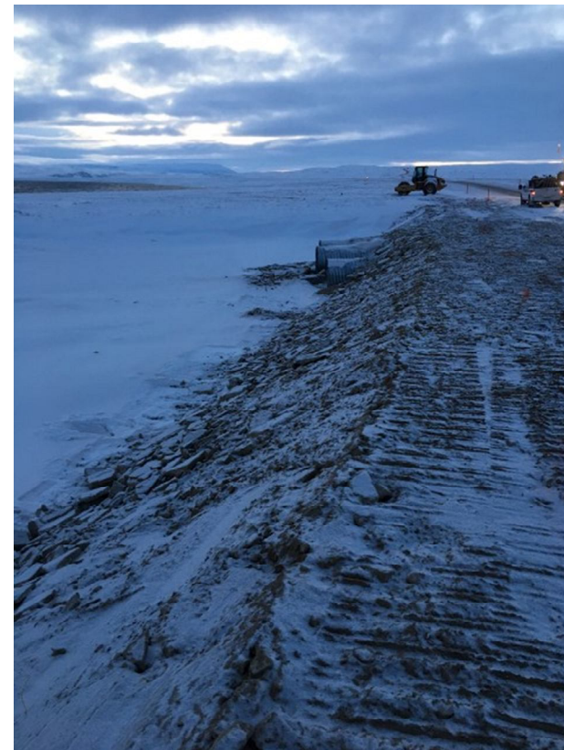
Figure 28. CV216 DS post-culvert extension 17-10-05
