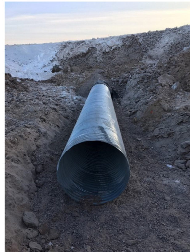
Figure 5. BG29 DS culvert extension installation 17-11-07
