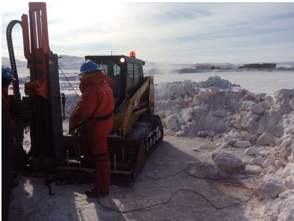
PHOTO 53 – Drilling Conditions at BH19-CPT19-15, April 2019
