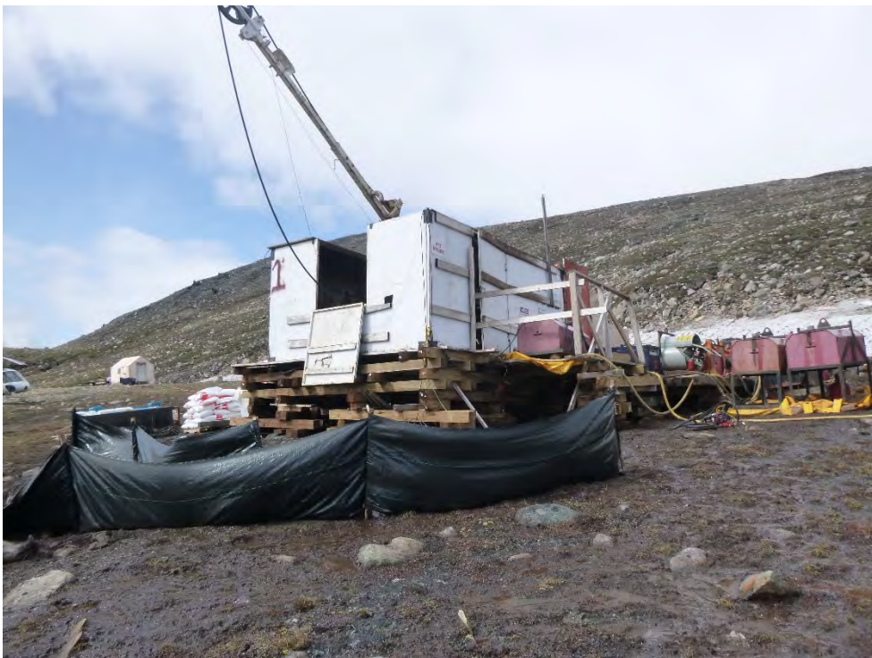
PHOTO 35 - Drilling Conditions at MR3-18-244, June 2019
