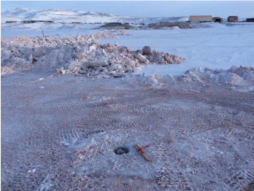
PHOTO 10 – Pre-Drilling Conditions at BH19-CPT19-01, April 2019
