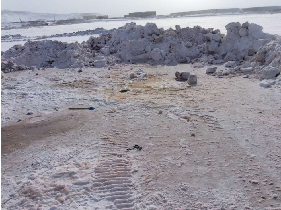
PHOTO 54 – Post-Drilling Conditions at BH19-CPT19-15, April 2019
