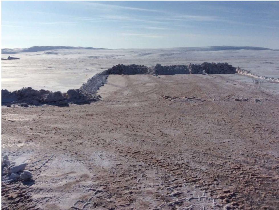
PHOTO 22 – Pre-Drilling Conditions at BH19-CPT19-05, April 2019
