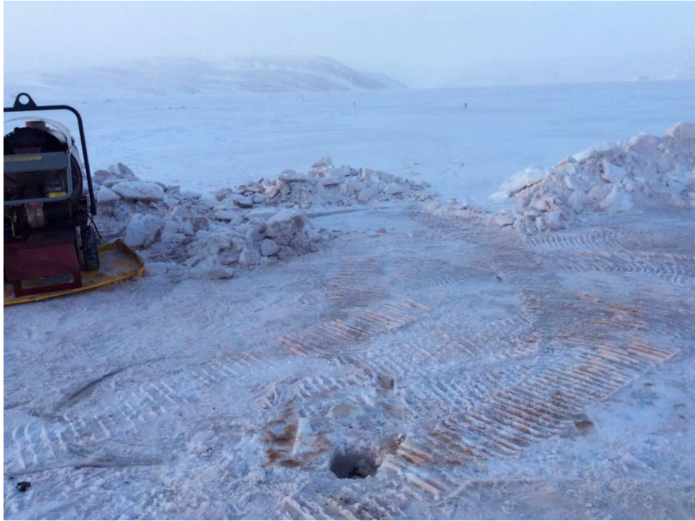
PHOTO 12 – Post-Drilling Conditions at BH19-CPT19-01, April 2019
