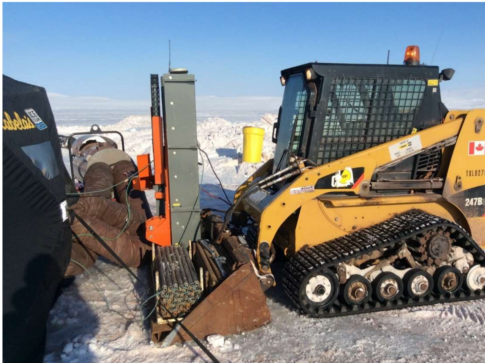
PHOTO 17 - Drilling Conditions at BH19-CPT19-03, April 2019
