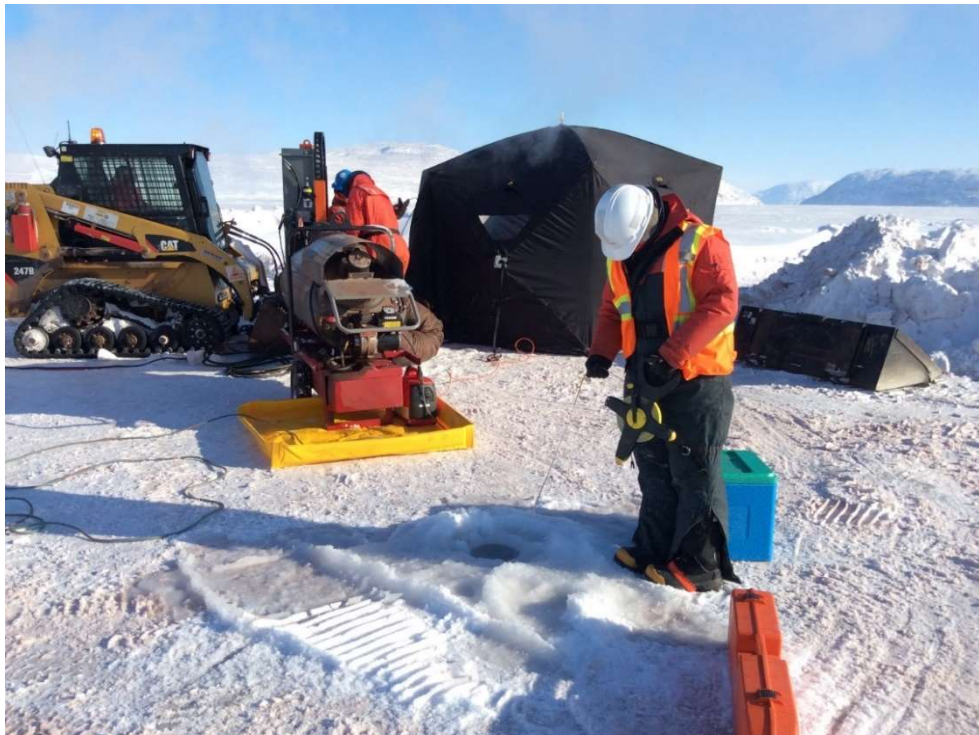
PHOTO 32 - Drilling Conditions at BH19-CPT19-08, April 2019
