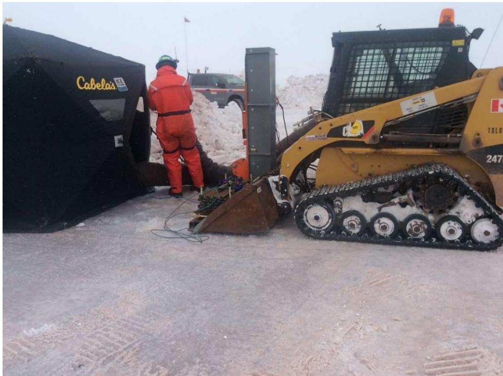
PHOTO 38 – Drilling Conditions BH19-CPT19-10, April 2019
