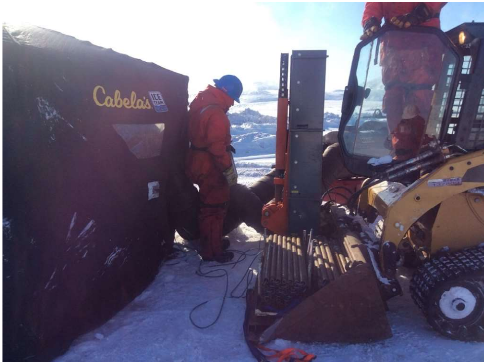
PHOTO 41 - Drilling Conditions at BH19-CPT19-11, April 2019
