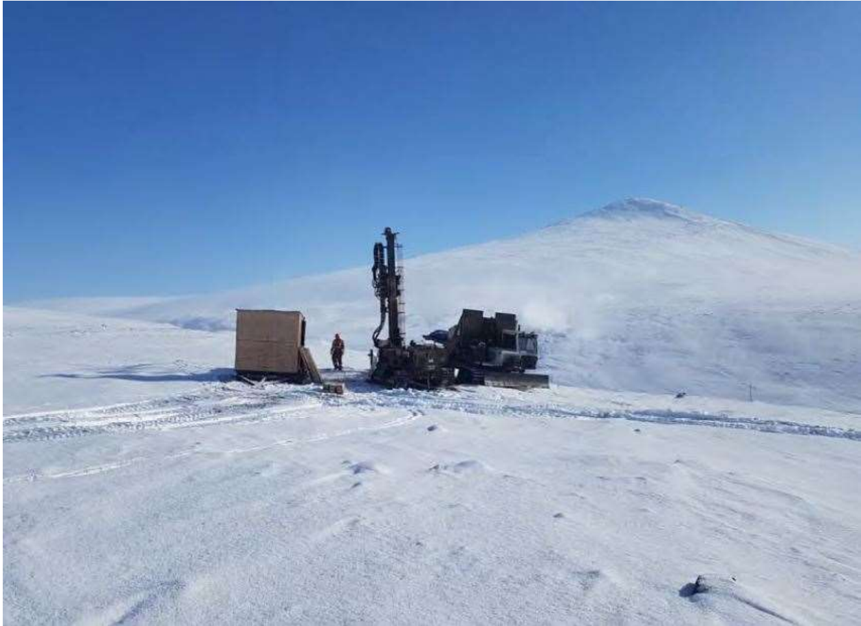
PHOTO 61 – Drilling Conditions at KM107-DH19-03, April 2019
