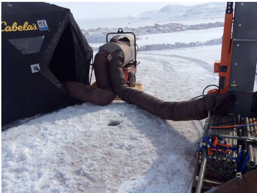
PHOTO 23 – Drilling Conditions at BH19-CPT19-05, April 2019
