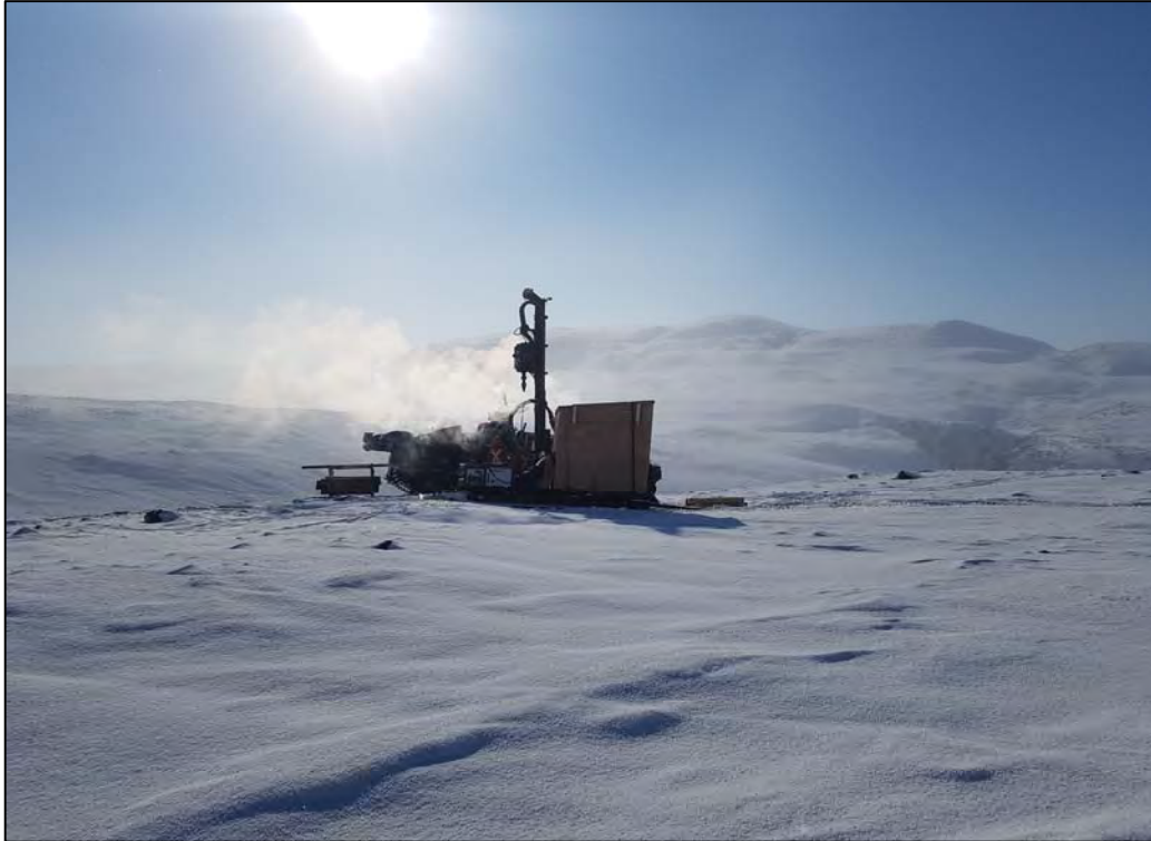
PHOTO 31 - KM107-DH19-03 Looking South During Drilling
