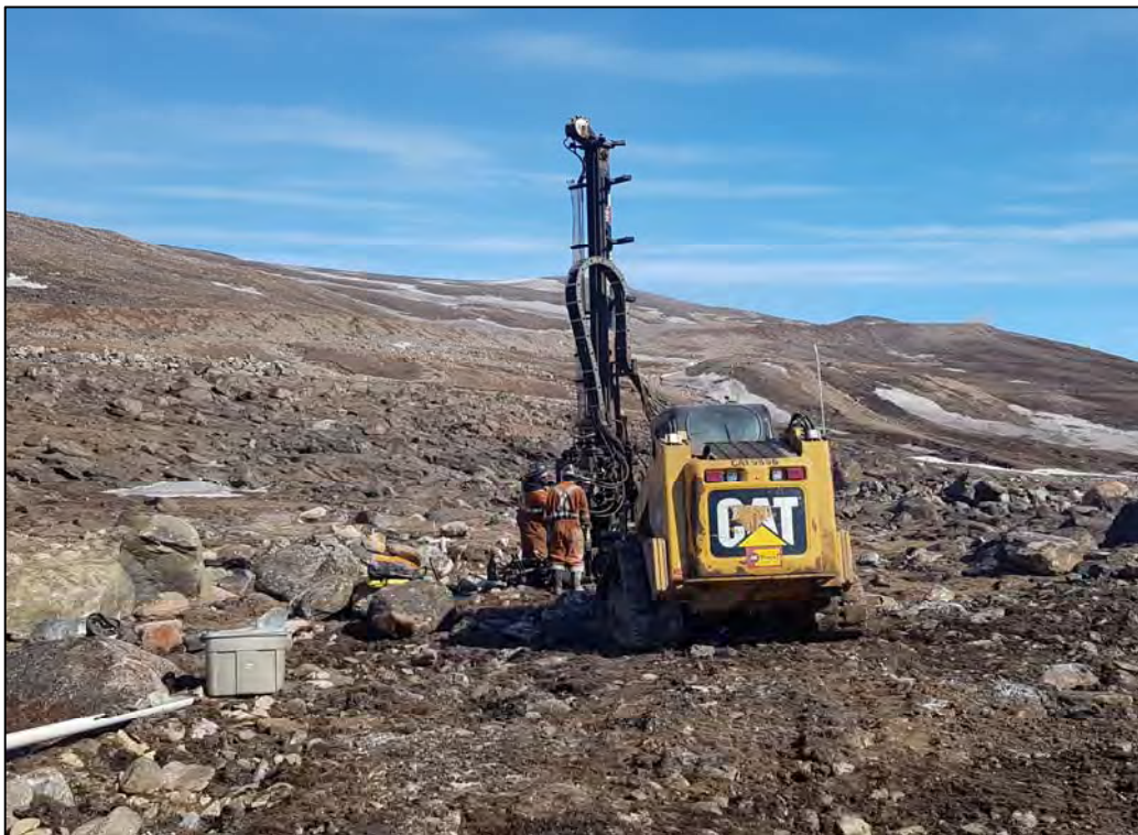
PHOTO 10 - KM106-DH19-03 Looking North During Drilling
