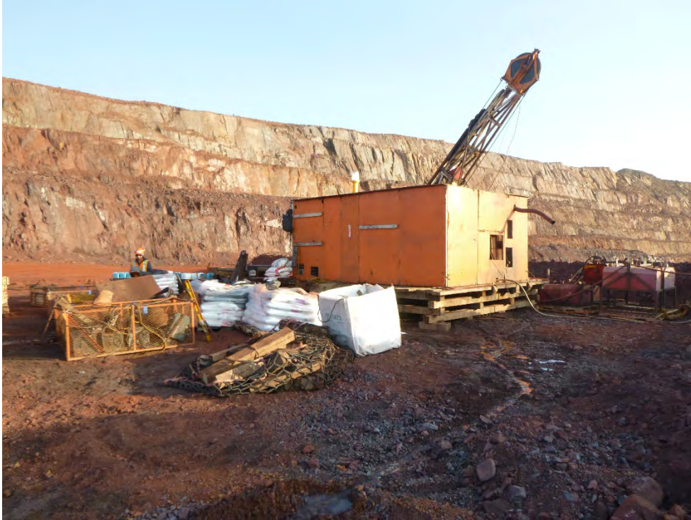
PHOTO 28 - Pre-Drilling Conditions at MR1-19-268, August 2019
