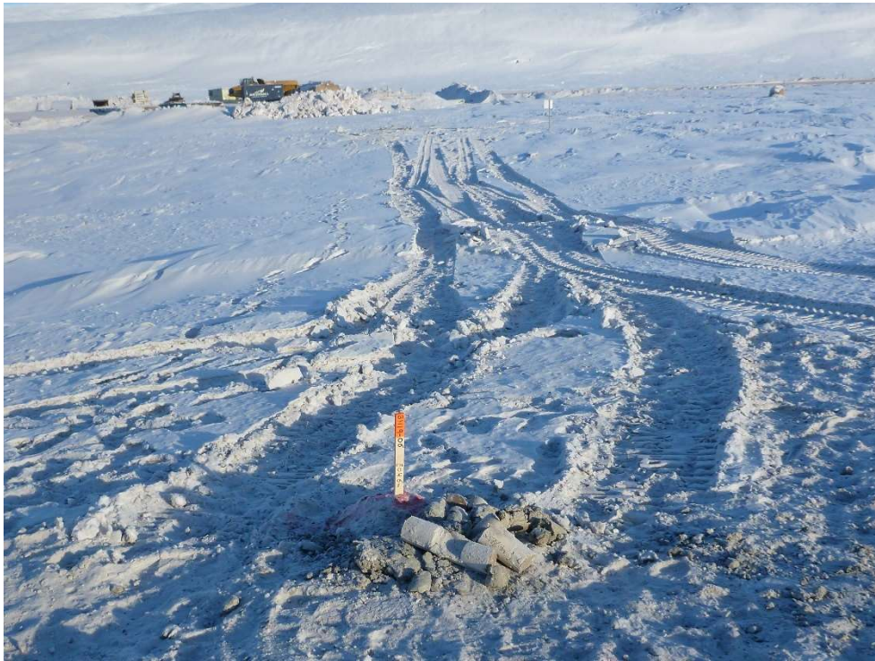
PHOTO 9 – Post-Drilling Conditions at BH19-06, February 2019
