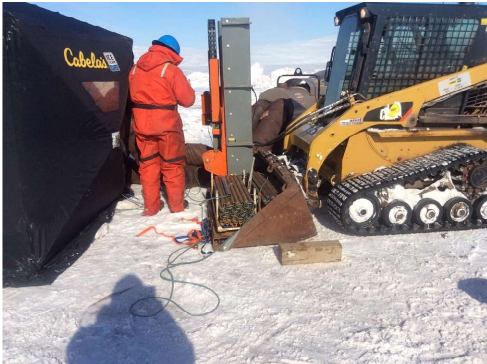
PHOTO 44 - Drilling Conditions at BH19-CPT19-12, April 2019
