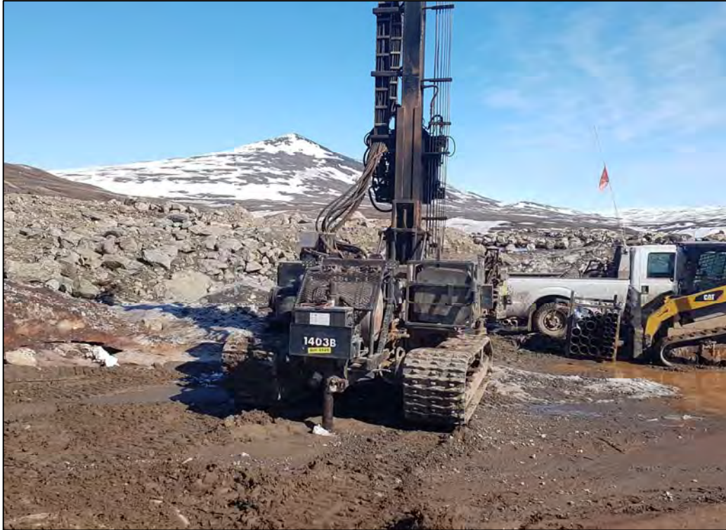
PHOTO 5 - KM106-DH19-02 Looking East During Drilling
