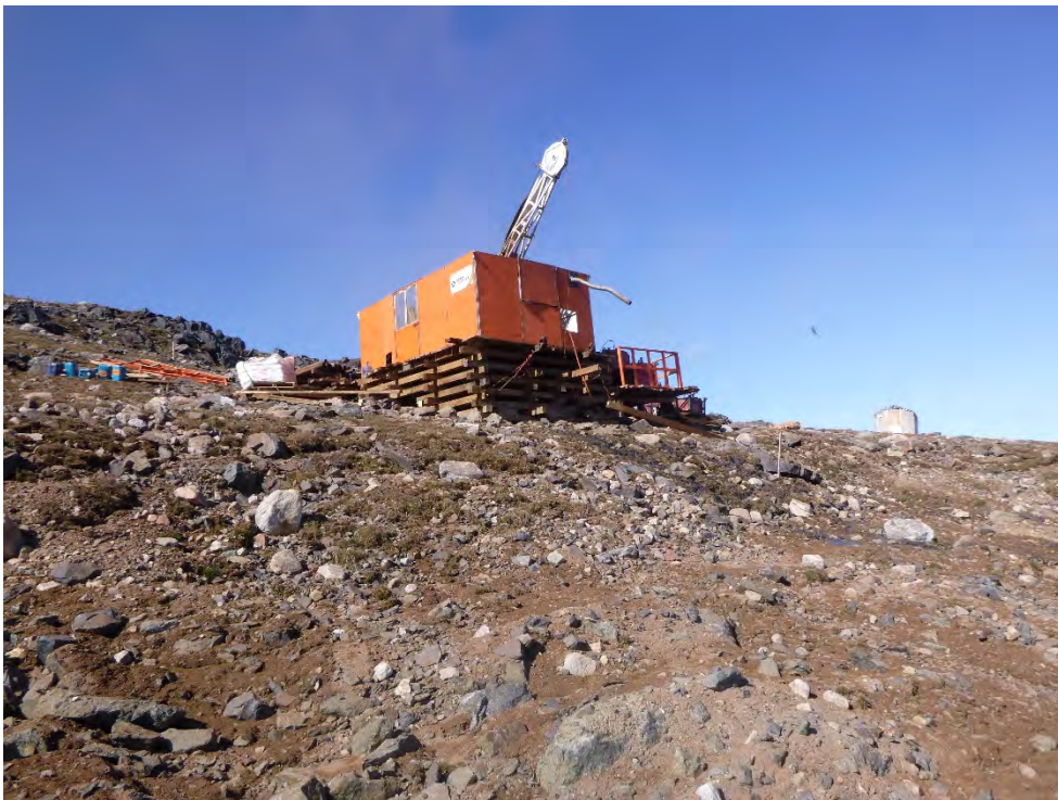
PHOTO 8 - Drilling Conditions at MR1-19-254, June 2019
