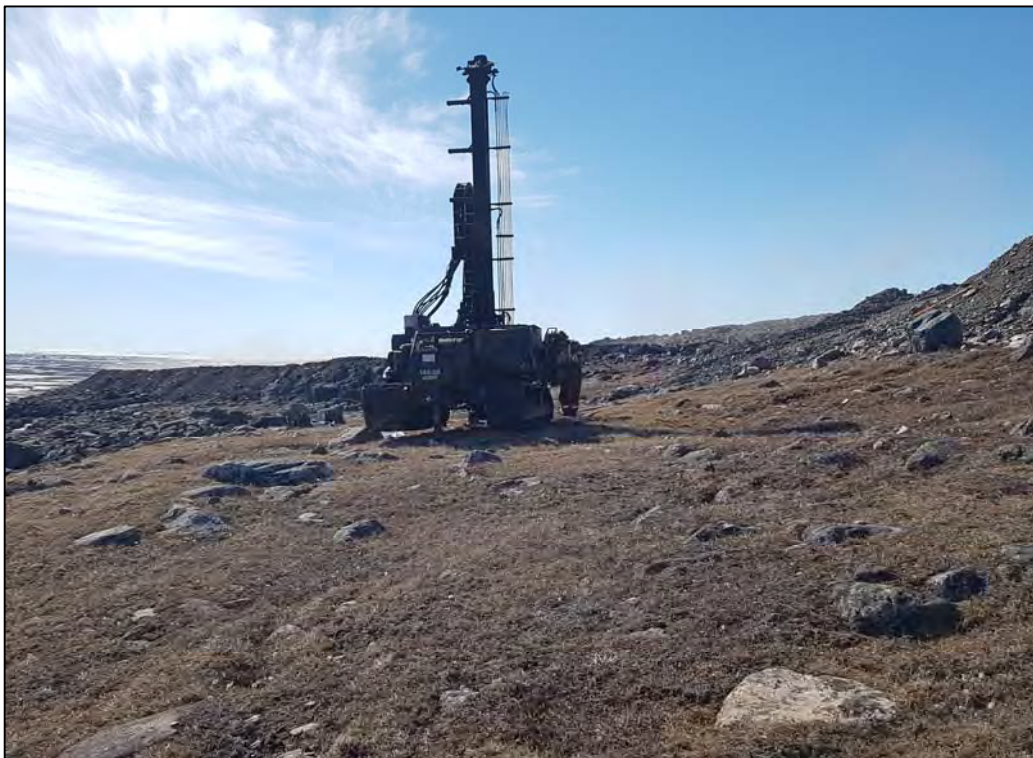
PHOTO 20 - KM106-DH19-05 Looking West During Drilling
