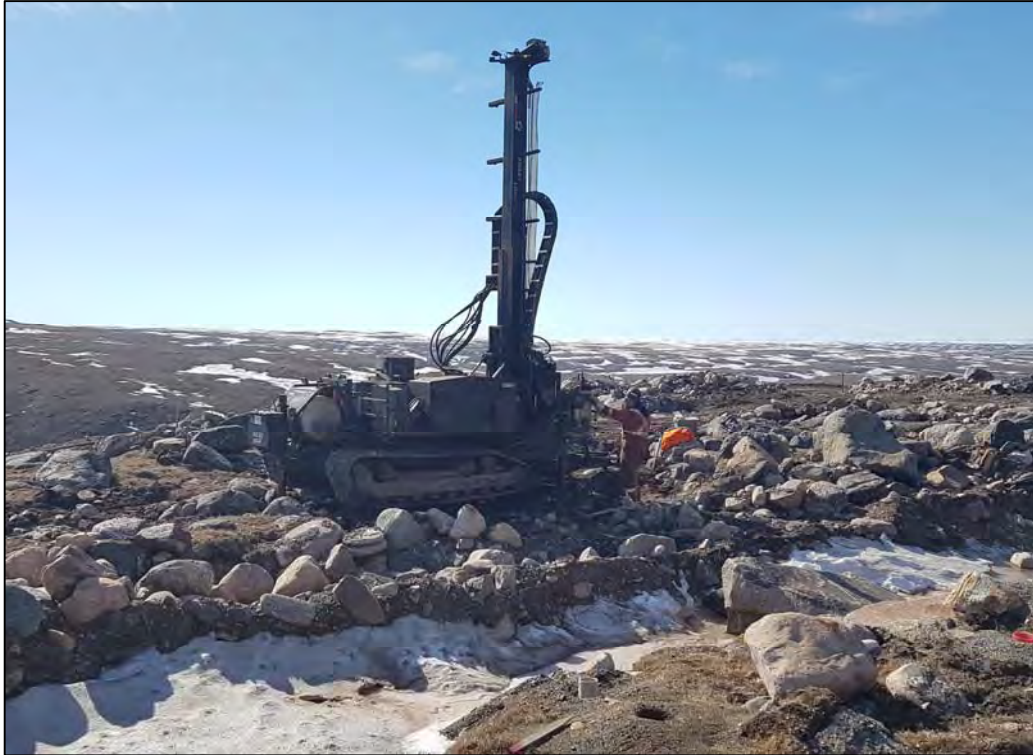
PHOTO 11 - KM106-DH19-03 Looking South During Drilling
