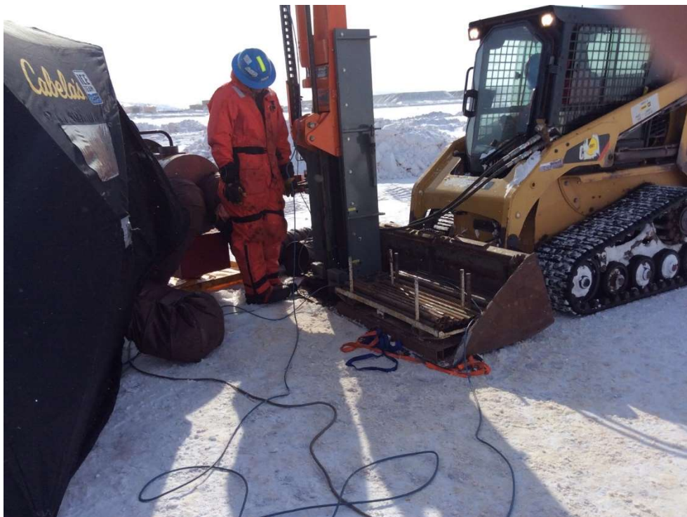
PHOTO 29 – Drilling Conditions at BH19-CPT19-07, April 2019
