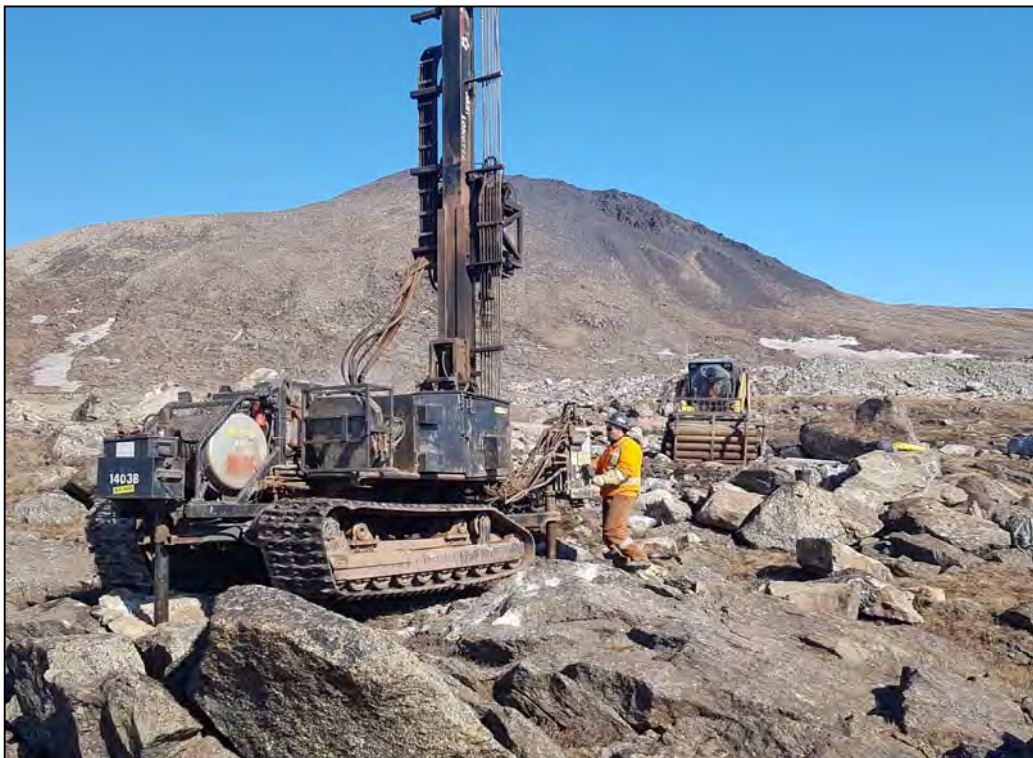
PHOTO 2 - KM106-DH19-01 Looking North During Drilling
