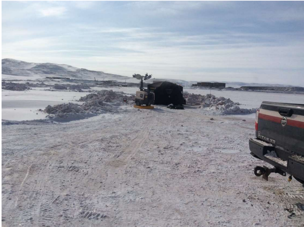
PHOTO 52 – Pre-Drilling Conditions at BH19-CPT19-15, April 2019
