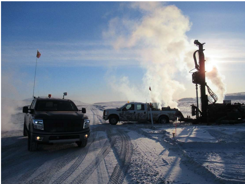
PHOTO 5 - Drilling Conditions at BH19-02, February 2019
