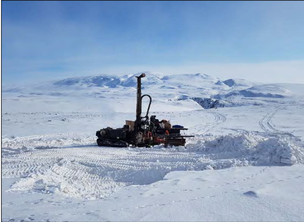
PHOTO 35 - KM107-DH19-04 Looking South During Drilling
