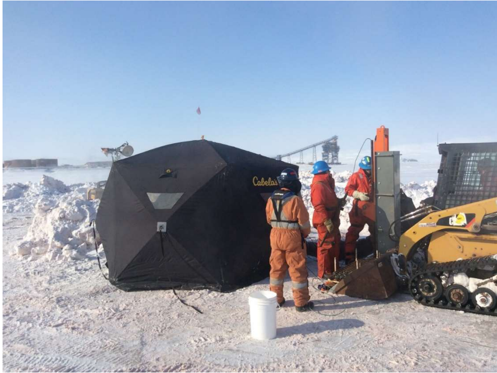
PHOTO 57 – Drilling Conditions at BH19-CPT19-17, April 2019
