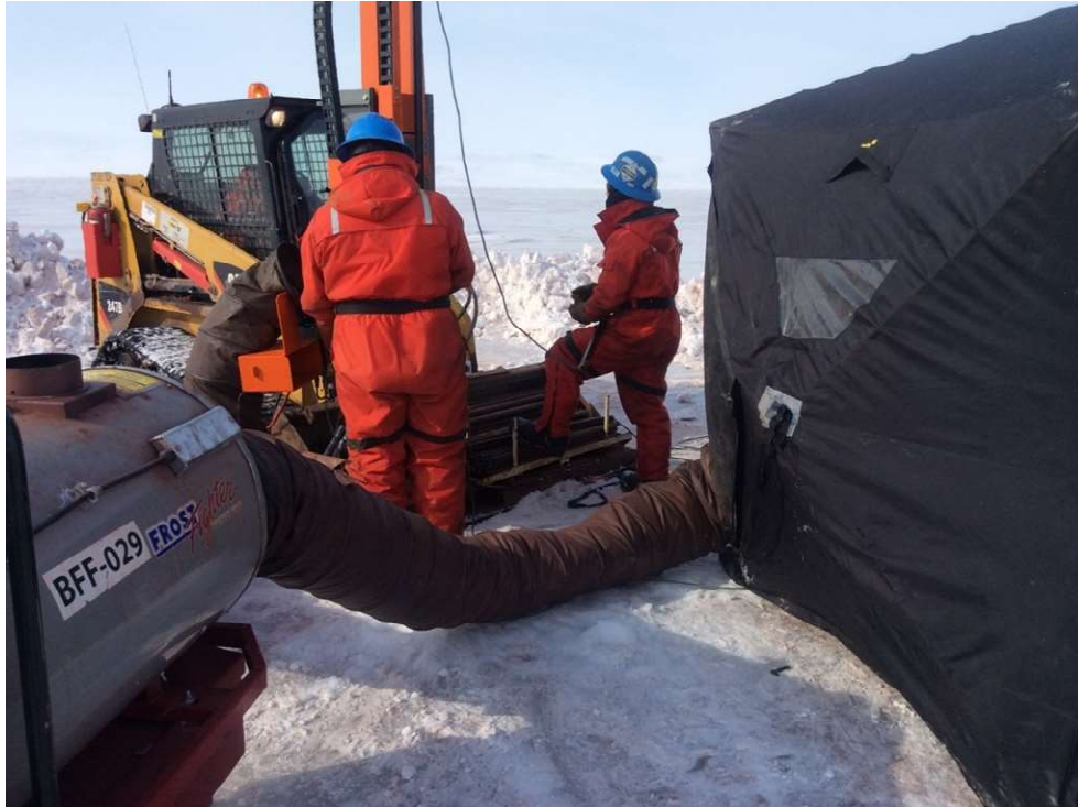
PHOTO 55 – Drilling Conditions at BH19-CPT19-16, April 2019
