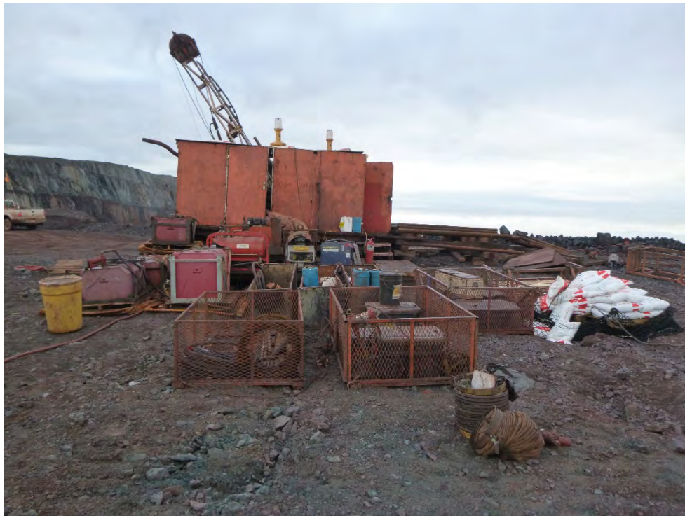
PHOTO 32 - Drilling Conditions at MR1-19-269, August 2019
