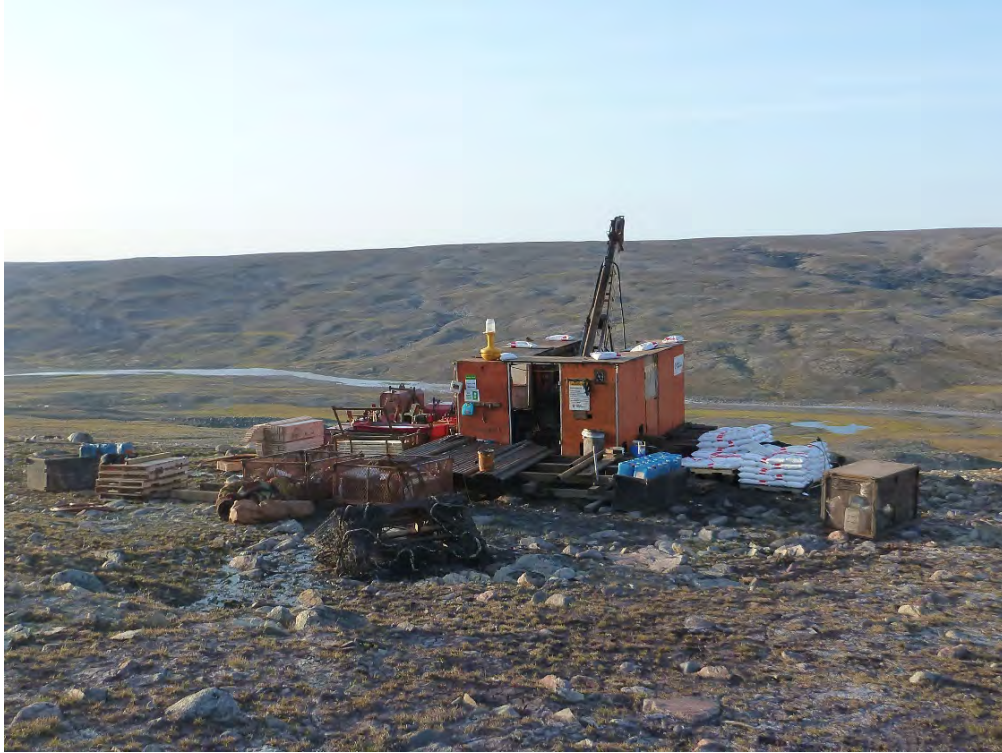
PHOTO 52 – Pre-Drilling Conditions at MR3-19-267, August 2019
