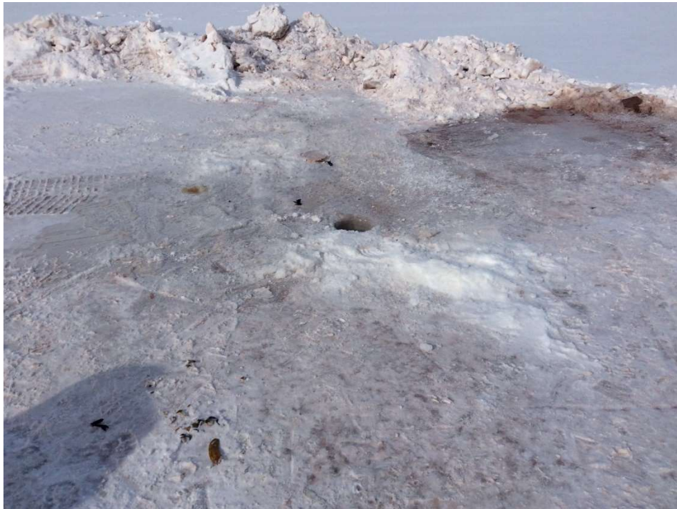
PHOTO 21 – Post-Drilling Conditions at BH19-CPT19-04, April 2019
