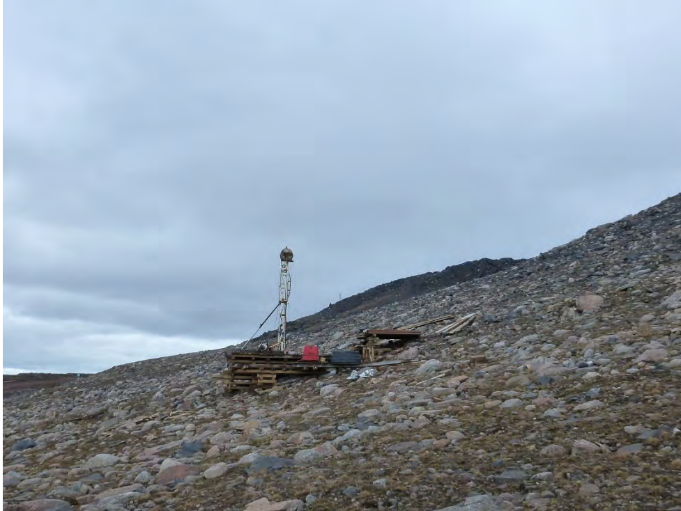
PHOTO 1 - Pre-Drilling Conditions at MR1-19-251, June 2019
