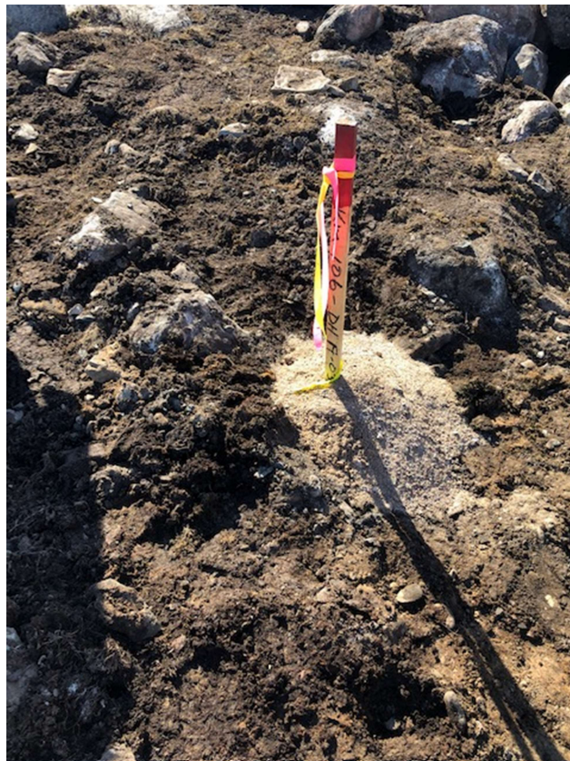
PHOTO 70 – Post Drilling Conditions at KM106-DH19-03, May 2019
