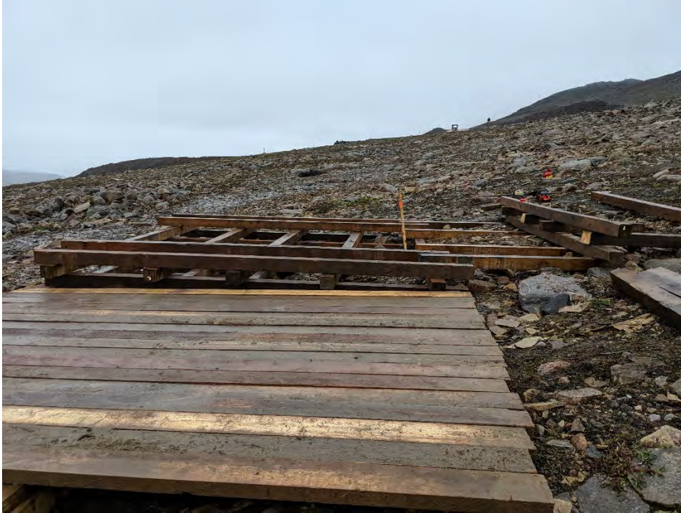
PHOTO 19 – Pre-Drilling Conditions at MR1-19-262, July 2019
