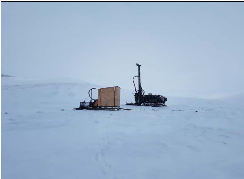
PHOTO 42 - KM107-DH19-06 Looking North During Drilling
