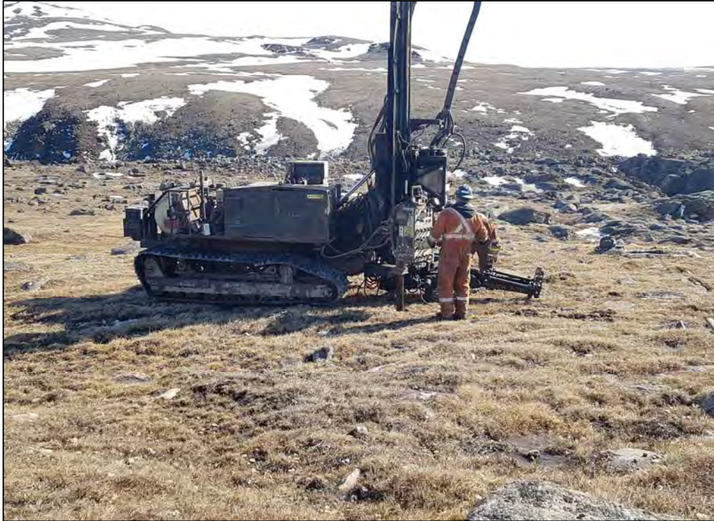
PHOTO 19 - KM106-DH19-05 Looking South During Drilling
