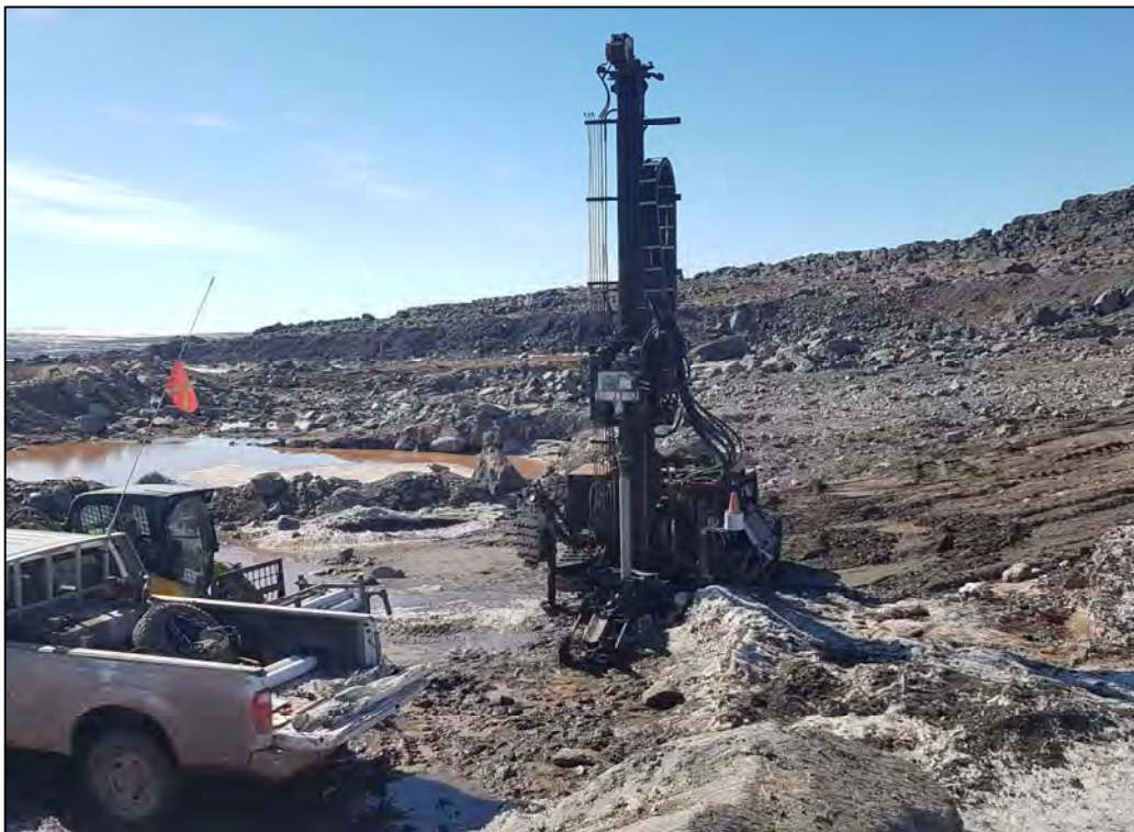
PHOTO 8 - KM106-DH19-02 Looking West During Drilling
