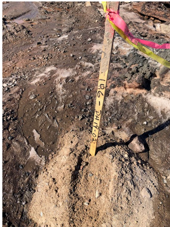
PHOTO 68 – Post Drilling Conditions at KM106-DH19-02, May 2019
