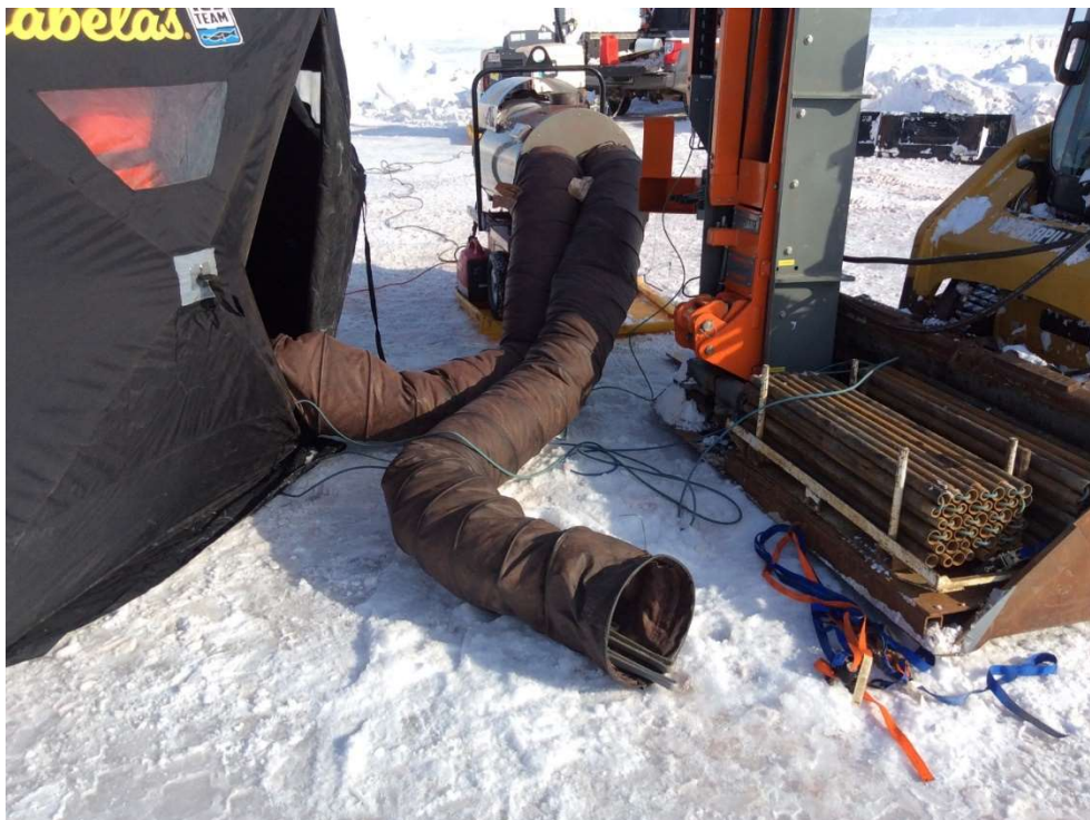
PHOTO 26 - Drilling Conditions at BH19-CPT19-06, April 2019
