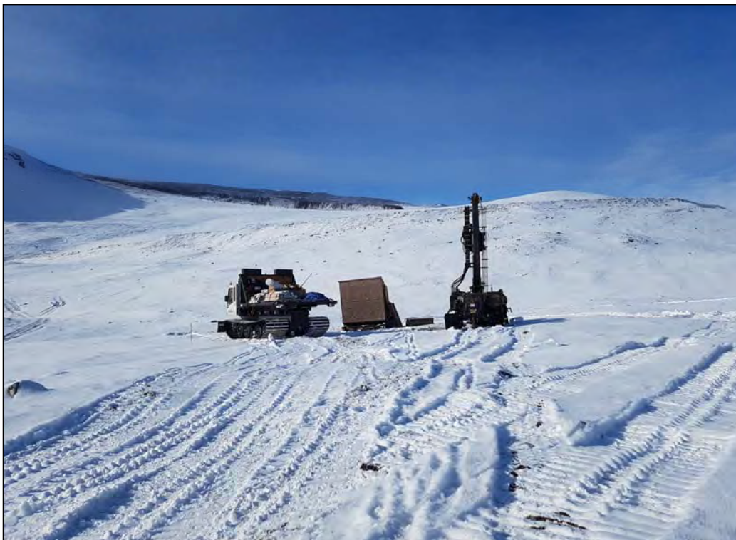
PHOTO 26 - KM107-DH19-02 Looking North During Drilling
