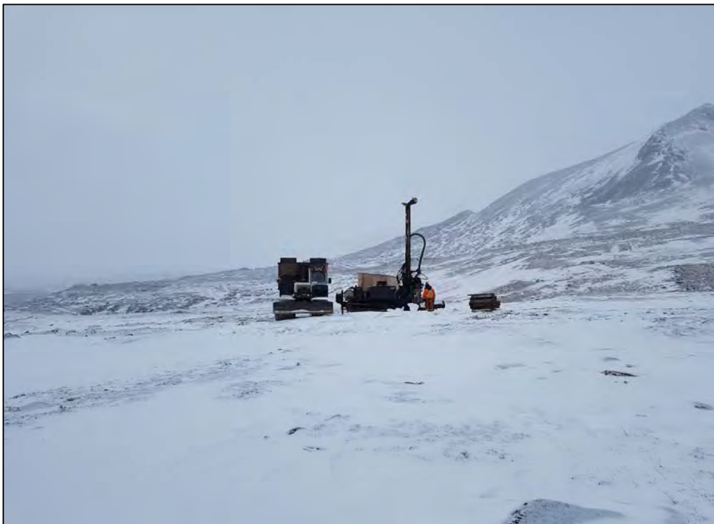
PHOTO 24 - KM107-DH19-01 Looking West During Drilling
