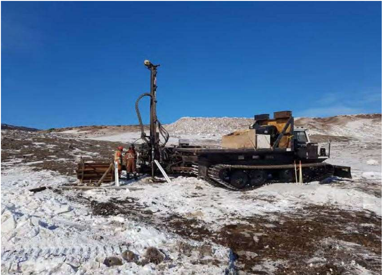
PHOTO 63 – Drilling Conditions at KM107-DH19-05, April 2019
