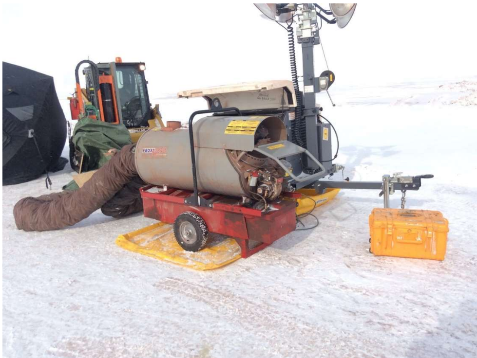
PHOTO 14 - Drilling Conditions at BH19-CPT19-02, April 2019
