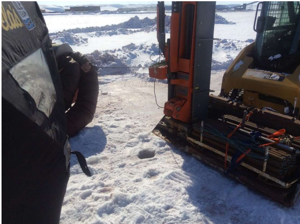
PHOTO 47 – Drilling Conditions at BH19-CPT19-13, April 2019
