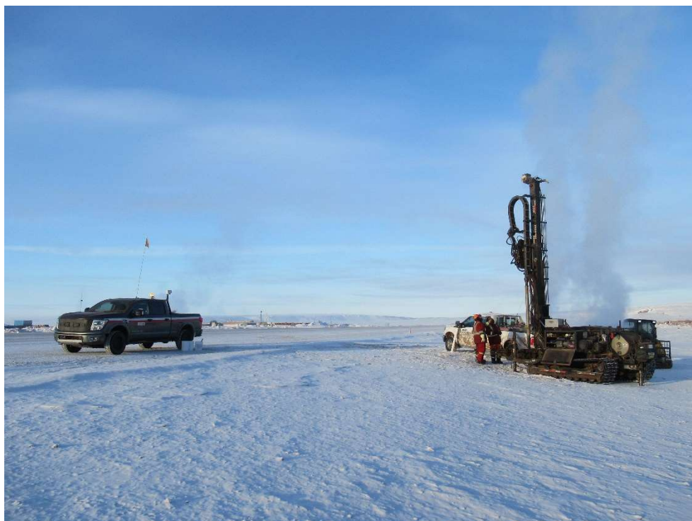
PHOTO 8 - Drilling Conditions at BH19-06, February 2019
