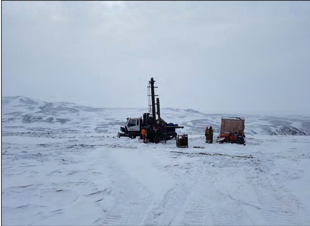
PHOTO 23 - KM107-DH19-01 Looking South During Drilling
