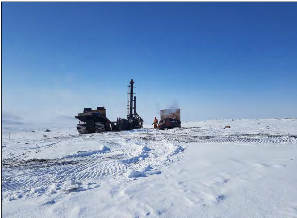
PHOTO 32 - KM107-DH19-03 Looking West During Drilling
