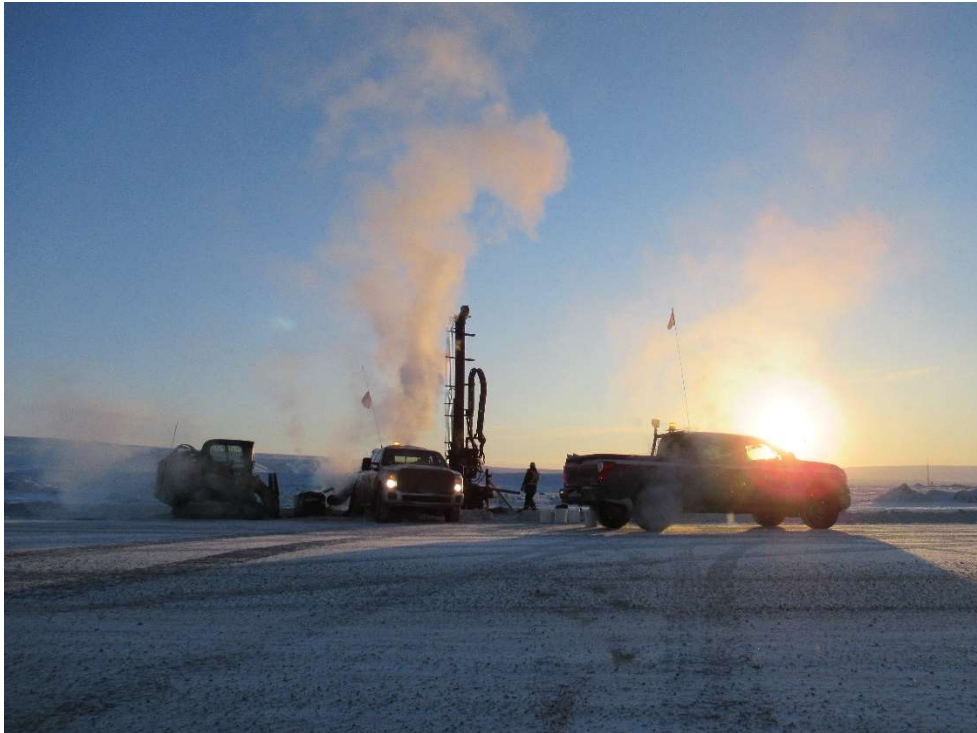
PHOTO 2 - Drilling Conditions at BH19-01, February 2019
