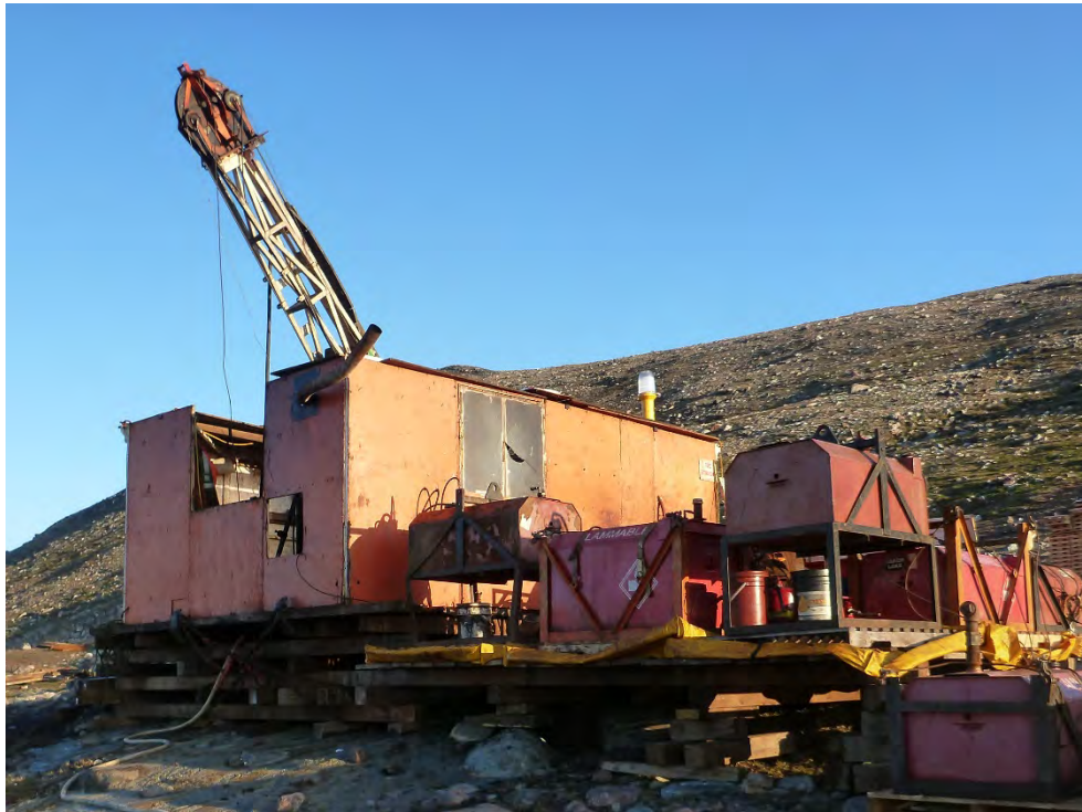
PHOTO 53 – Drilling Conditions at MR3-19-267, August 2019
