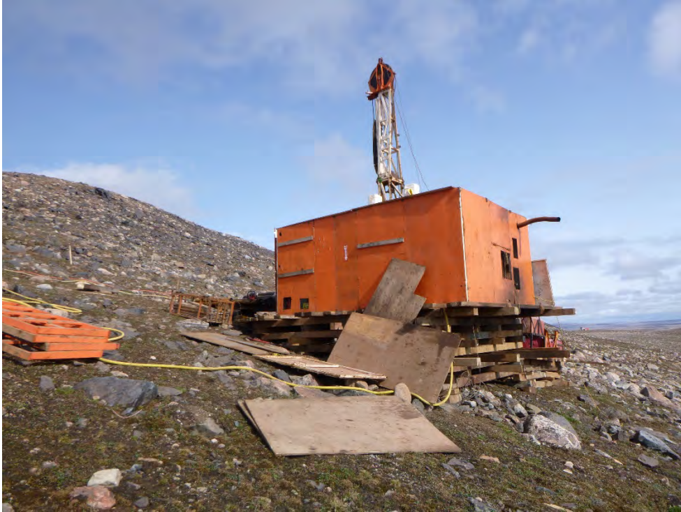
PHOTO 16 - Pre-Drilling Conditions at MR1-19-260, July 2019
