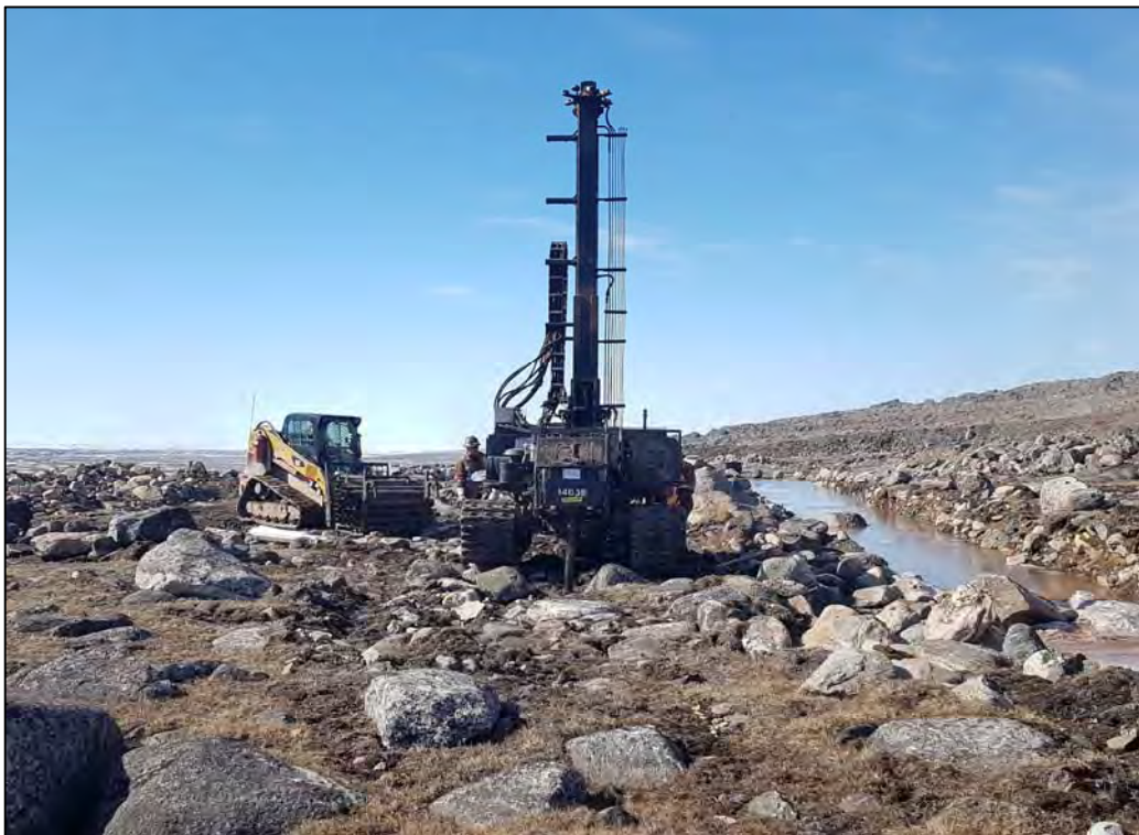
PHOTO 12 - KM106-DH19-03 Looking West During Drilling
