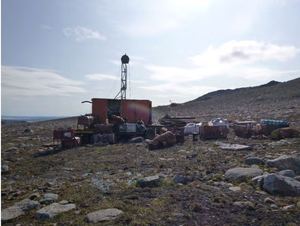
PHOTO 22 – Pre-Drilling Conditions at MR1-19-264, July 2019
