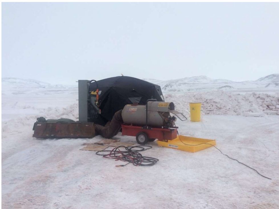
PHOTO 35 - Drilling Conditions BH19-CPT19-09, April 2019
