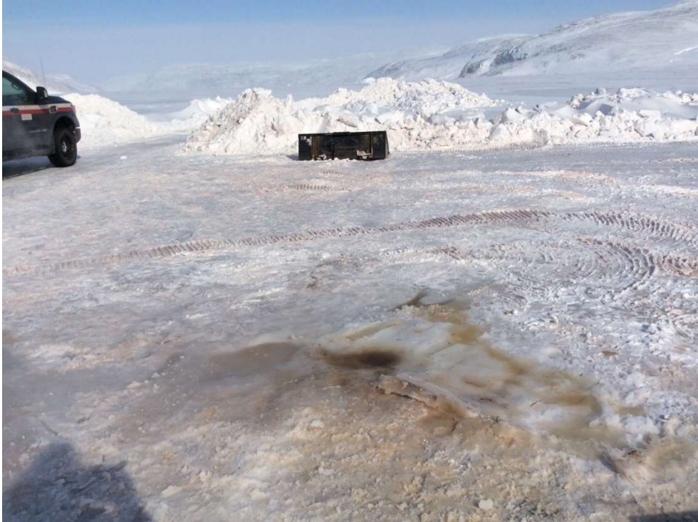
PHOTO 27 – Post-Drilling Conditions at BH19-CPT19-06, April 2019
