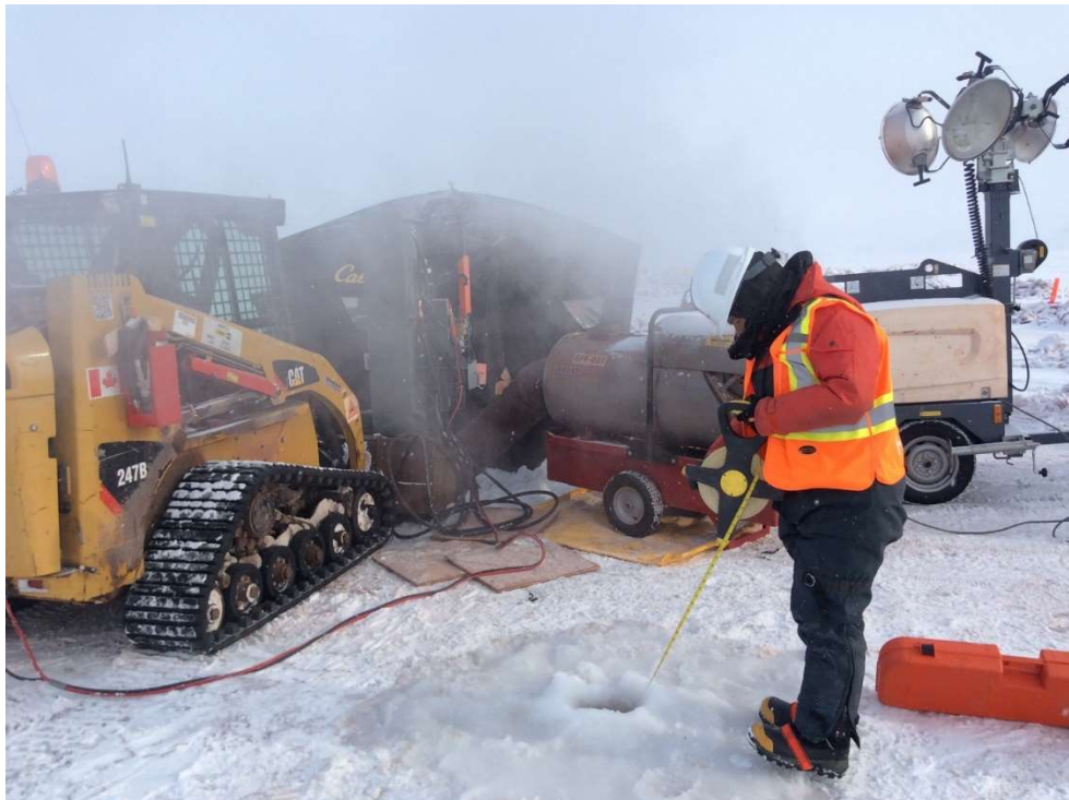
PHOTO 20 - Drilling Conditions at BH19-CPT19-04, April 2019
