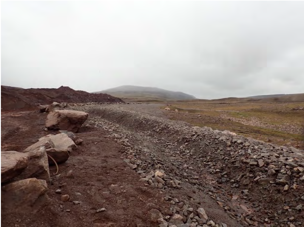
Photo 7. July 11 th , 2019 – Dry collection ditch.
