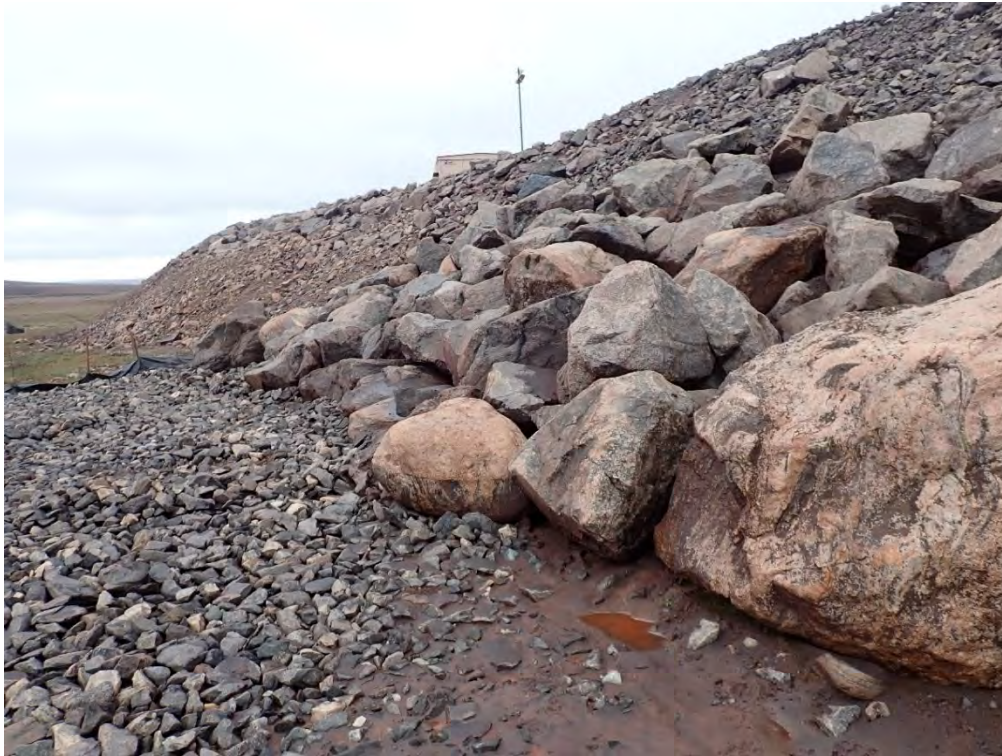
Photo 9. July 11 th , 2019 – CP-SEEPAGE-1 sample location.
