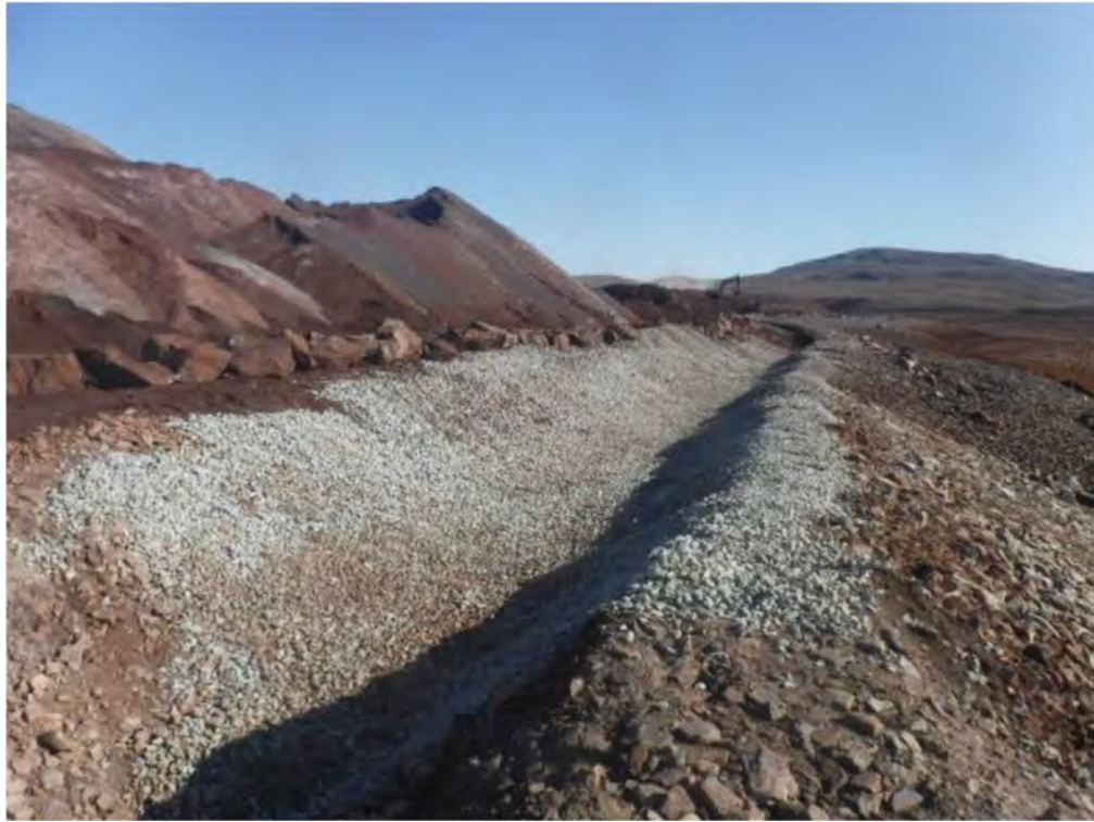
Photo 5. September 3 rd , 2019 – Crusher Facility ditch repairs.
