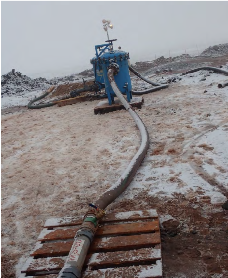
Photo 3. September 30 th , 2019 – Bag Filters Installed.
