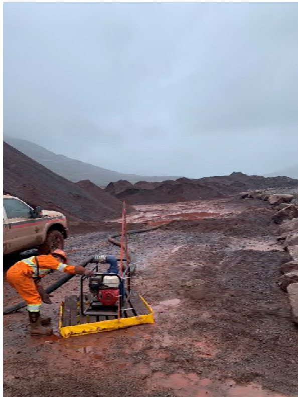
Photo 5. July 10 th , 2019 – Pump set up to bypass ditch.
