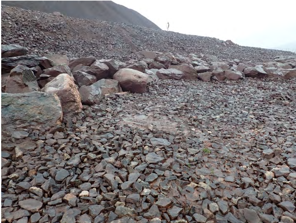
Photo 3. July 10 th , 2019 – CP-SEEPAGE-1 sample location.
