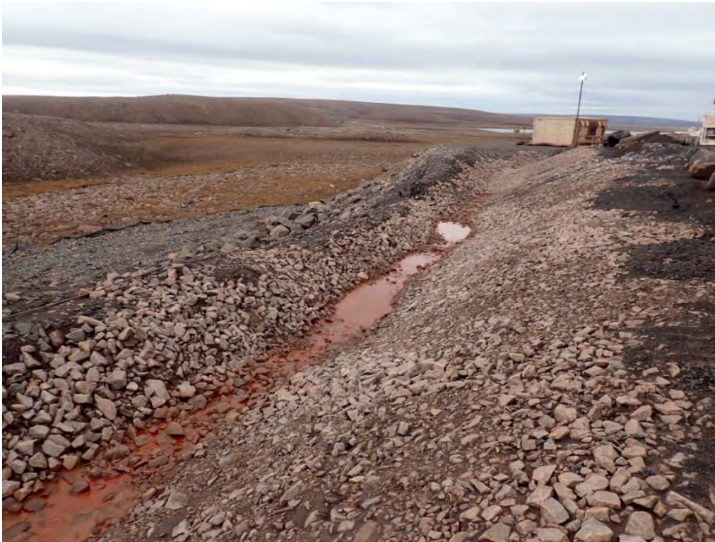
Photo 1. August 31 st , 2019 – Crusher Facility runoff into ditch.
