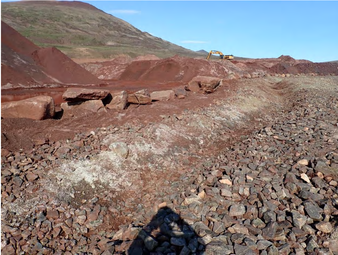
Photo 1. July 8 th , 2019 – Dry collection ditch.
