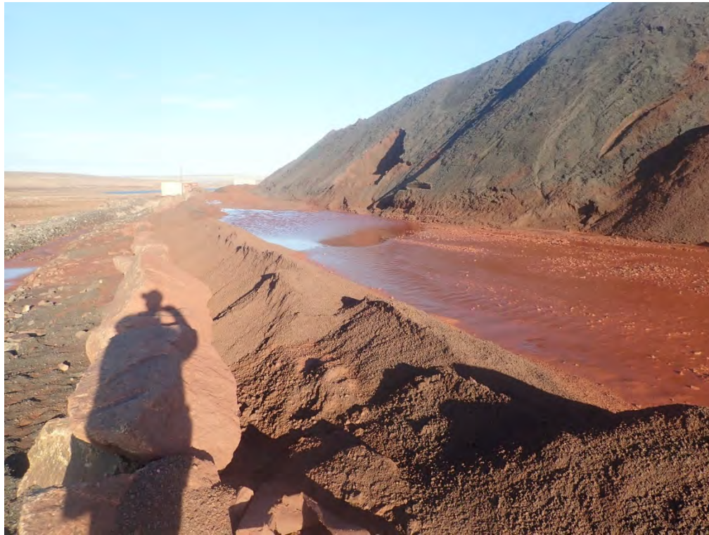
Photo 3. September 1 st , 2019 – Crusher Facility runoff berm.
