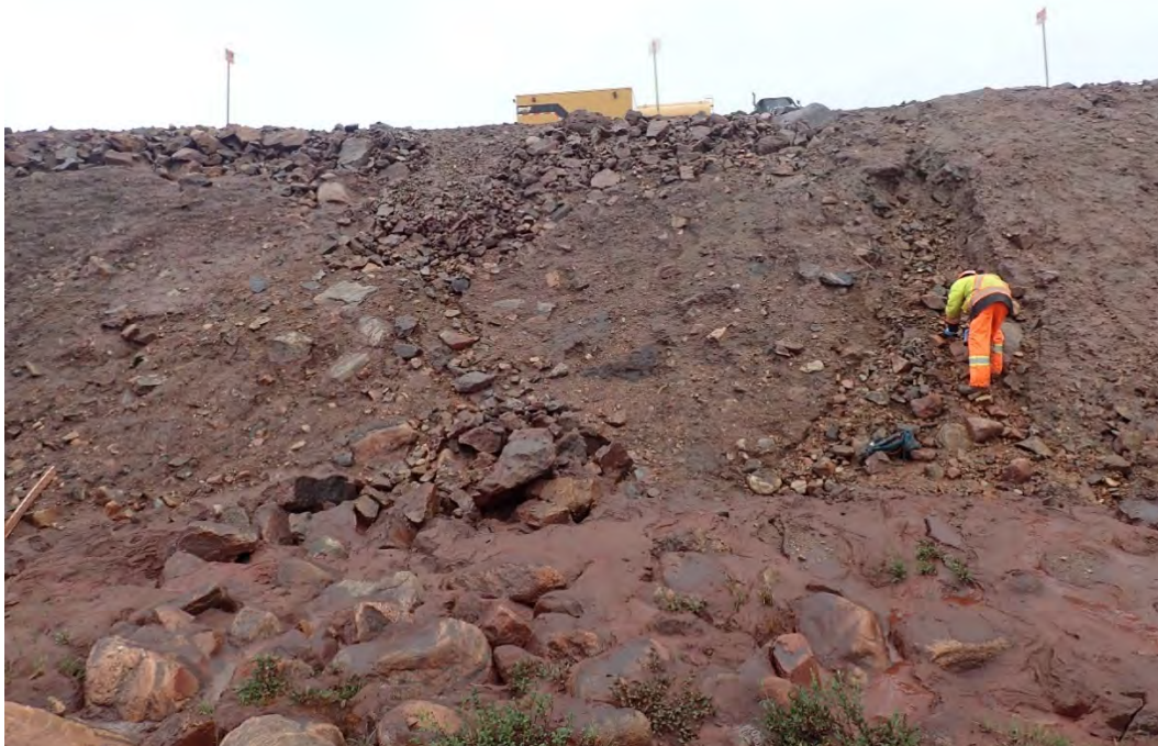
Photo 10. July 11 th , 2019 – CP-SEEPAGE-2 sample location.
