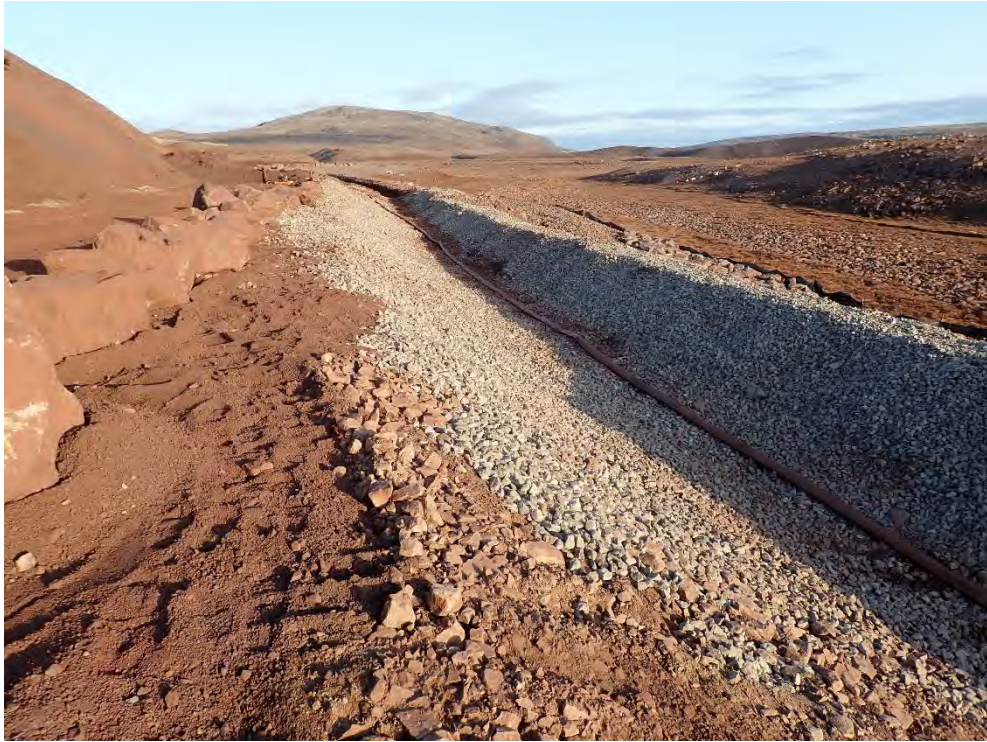
Photo 9. September 14 th , 2019 – Crusher Facility pump set up to bypass ditch.
