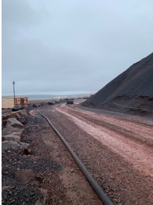
Photo 6. July 10 th , 2019 – Pump set up to bypass ditch.
