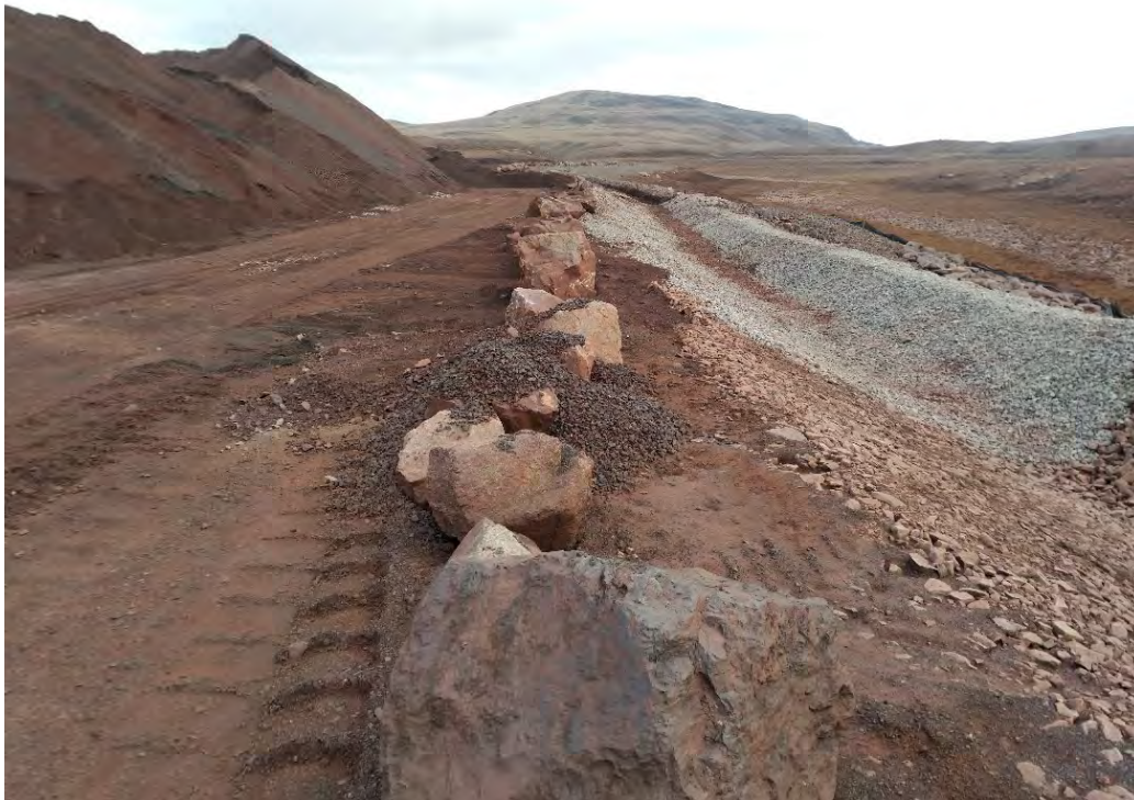
Photo 8. September 12 th , 2019 – Crusher Facility ditch dry.
