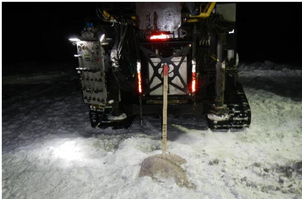
PHOTO 6 – Post-Drilling Conditions at BH16-B002
