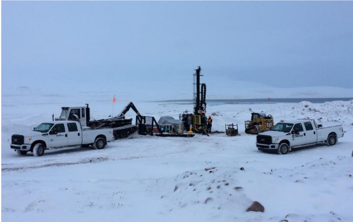
PHOTO 1 – Geotechnical Drilling Set Up, October 2016
