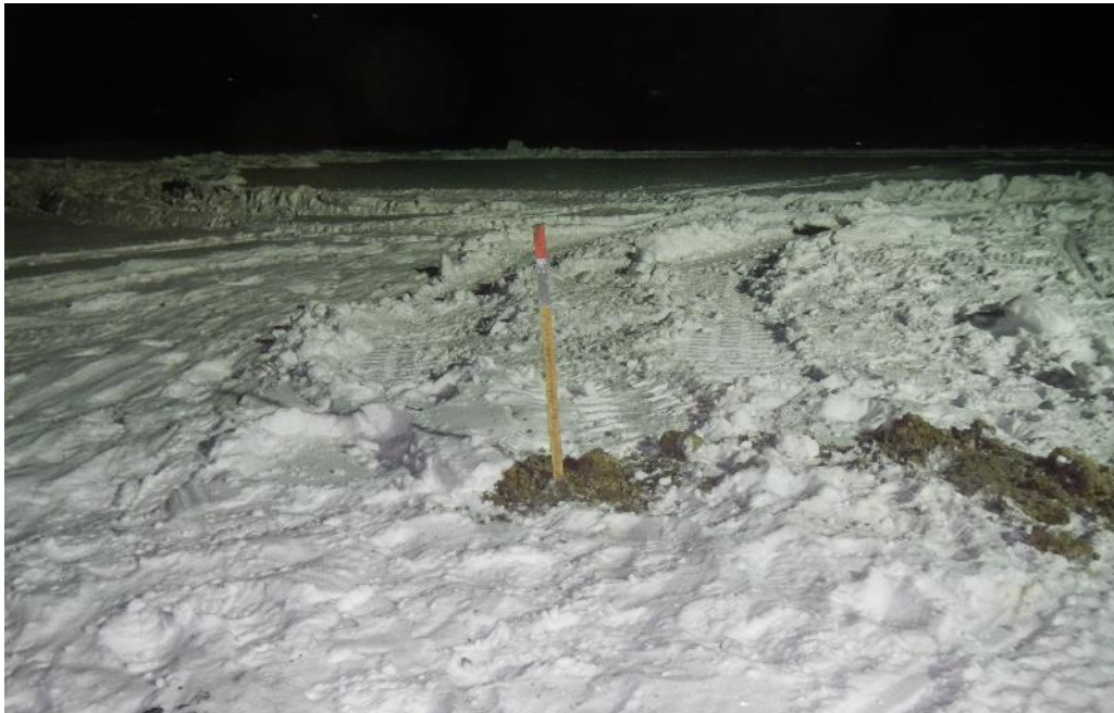
PHOTO 4 – Post-Drilling Site Conditions at BH16-C017
