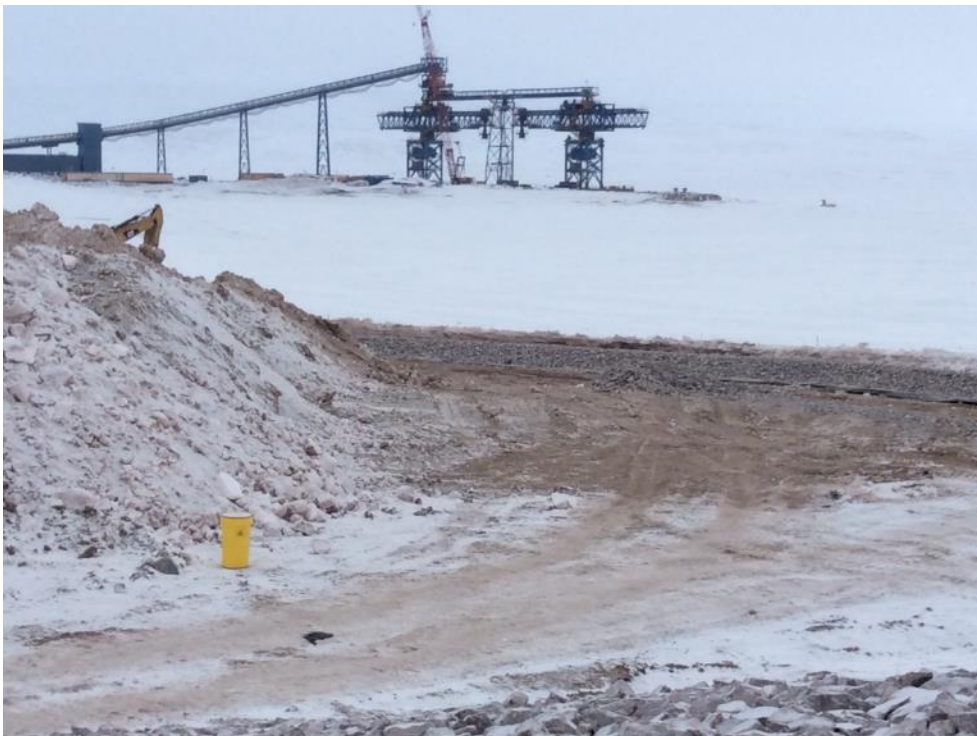
Photo 4 - Spill kit location for the snow/sand containment berm construction, 12 April 2019
