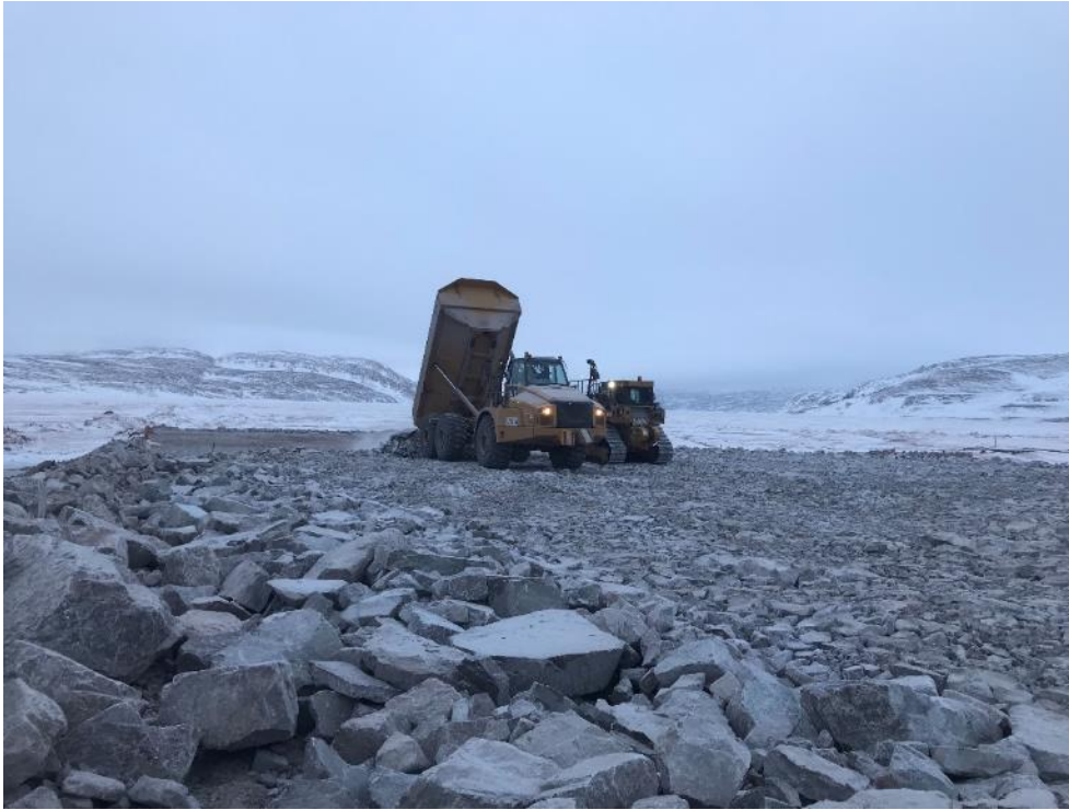
Photo 17 - Rock placement on the Freight Dock causeway (looking north), 3 May 2019
