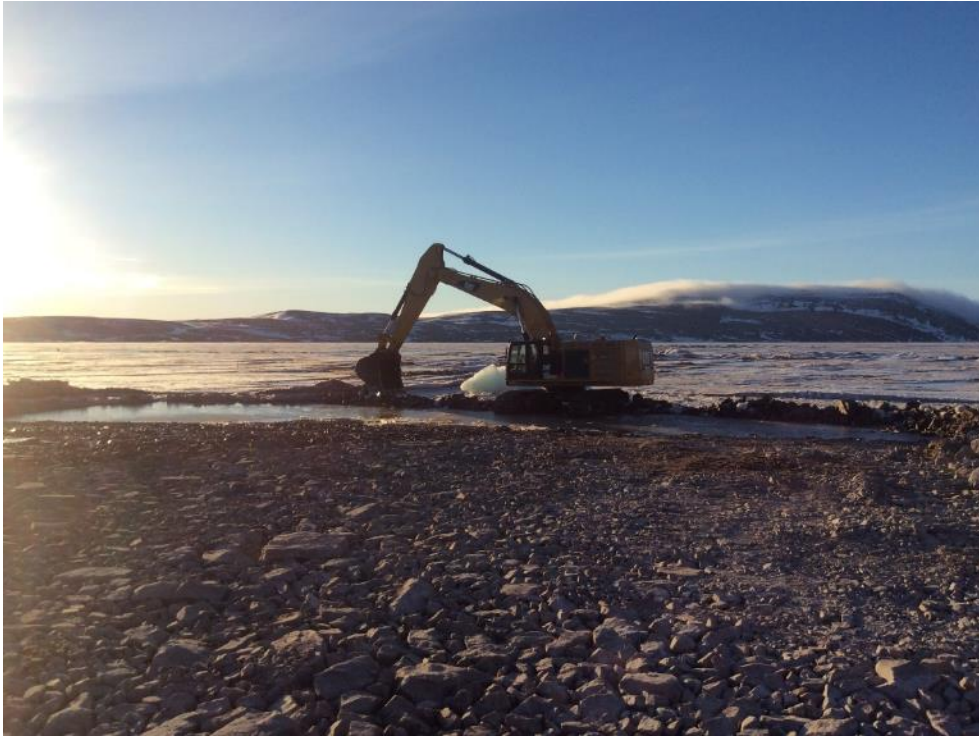
Photo 23 - Ice breaking and removal with a 374 excavator at high tide, 13 May 2019
