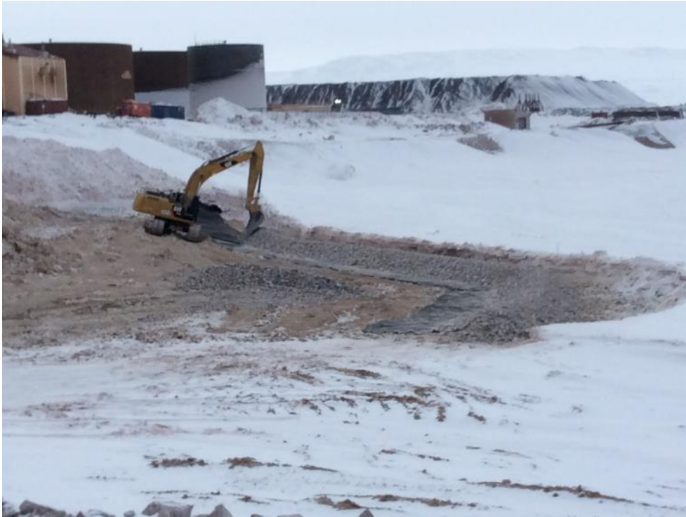
Photo 3 - Construction of the snow/sand containment berm (looking west), 12 April 2019
