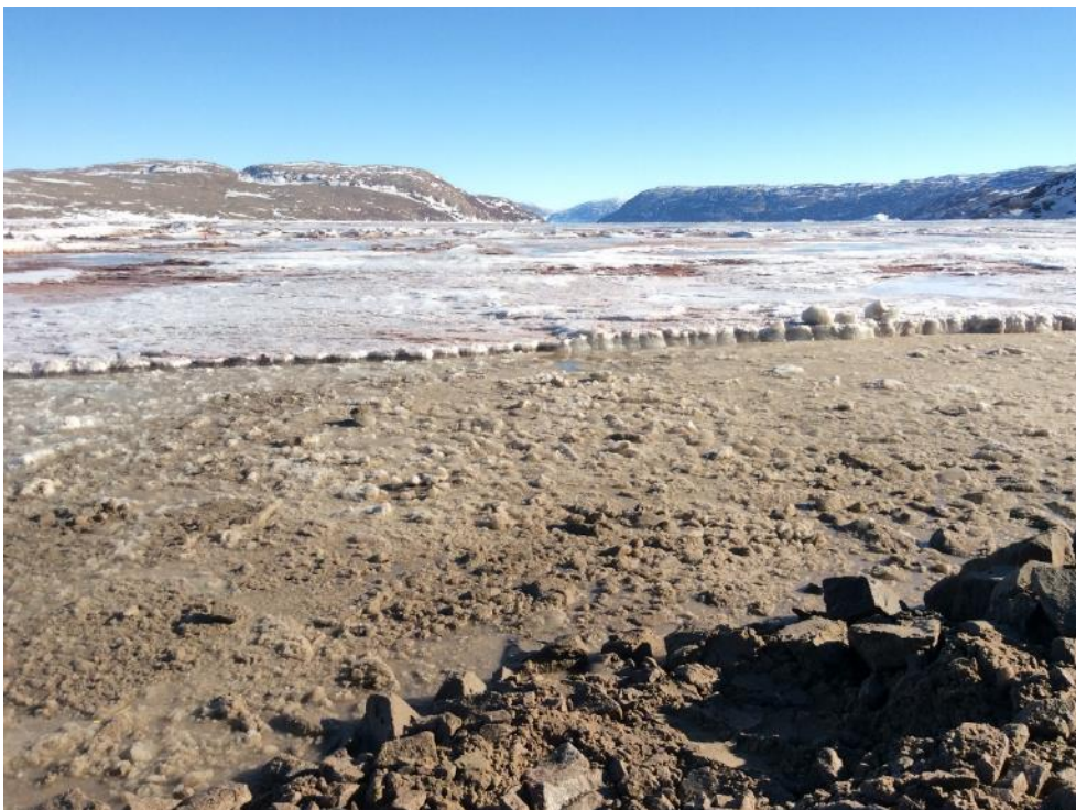
Photo 26 - Turbidity being contained within ice and slush on the water surface during dredging activities with an excavator, 16 May 2019
