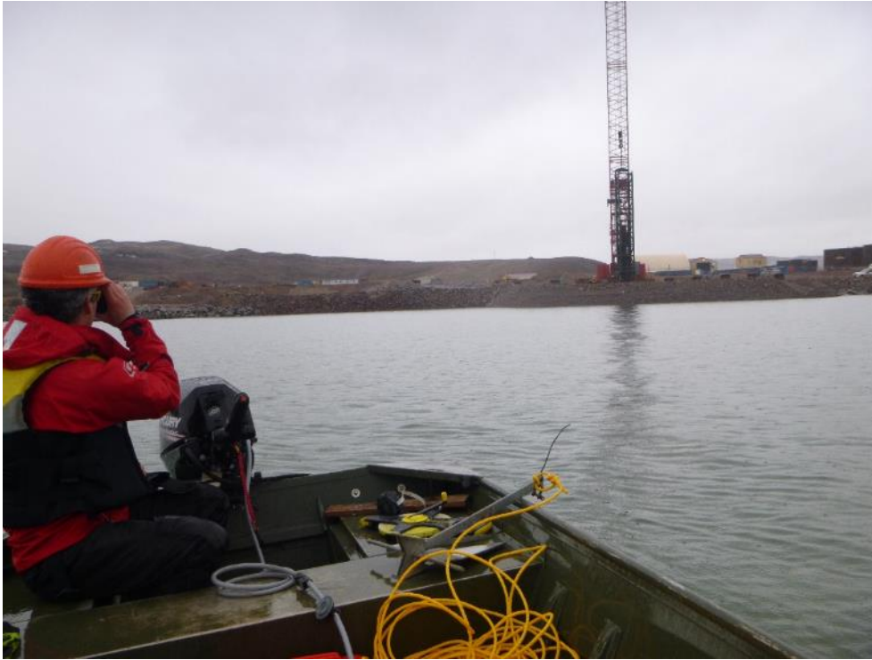
Photo 41 - Monitoring of construction activities during impact pile driving, 18 June 2019
