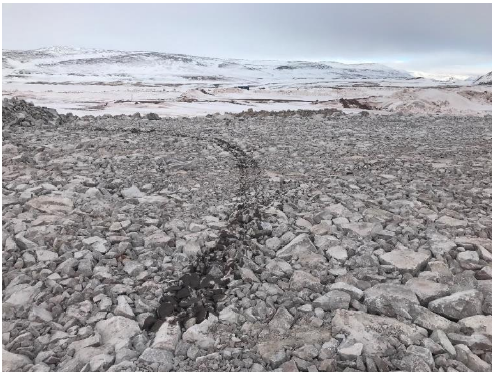
Photo 18 - Spill of hydraulic fluids on the Freight Dock, approximately 120 m from the causeway entrance (looking south), 3 May 2019
