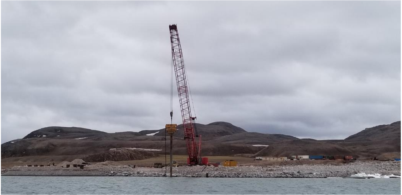
Photo 43 - Placement of the mooring piles (looking southwest), 20 June 2019
