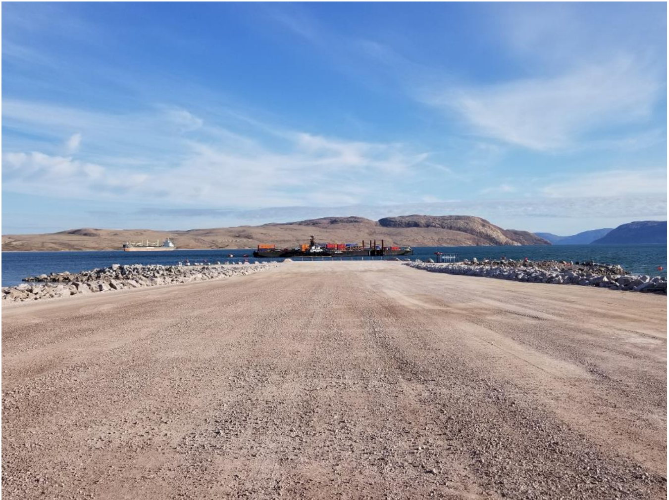
Photo 62 - View of the Freight Dock following construction and removal of equipment (looking north), 11 August 2019
