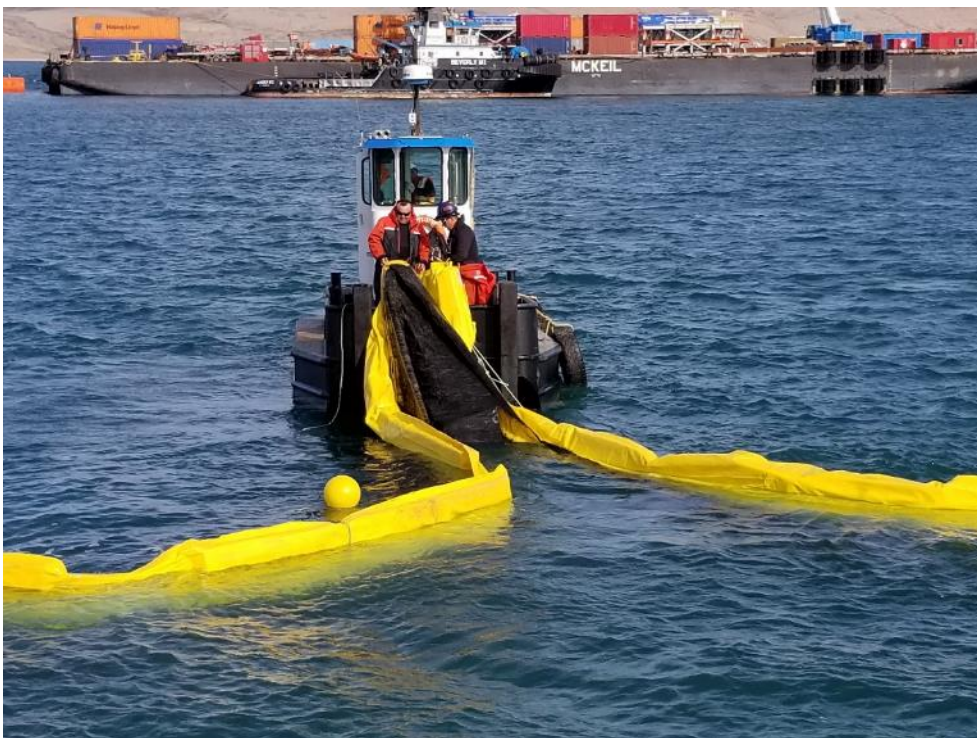
Photo 60 - Lifting of the silt curtain during removal, 10 August 2019
