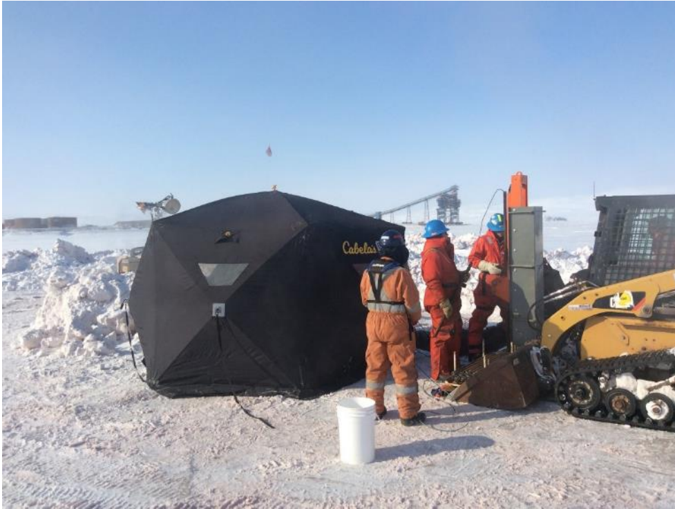
Photo 11 - ConeTec conducting geotechnical CPT testing, 25 April 2019
