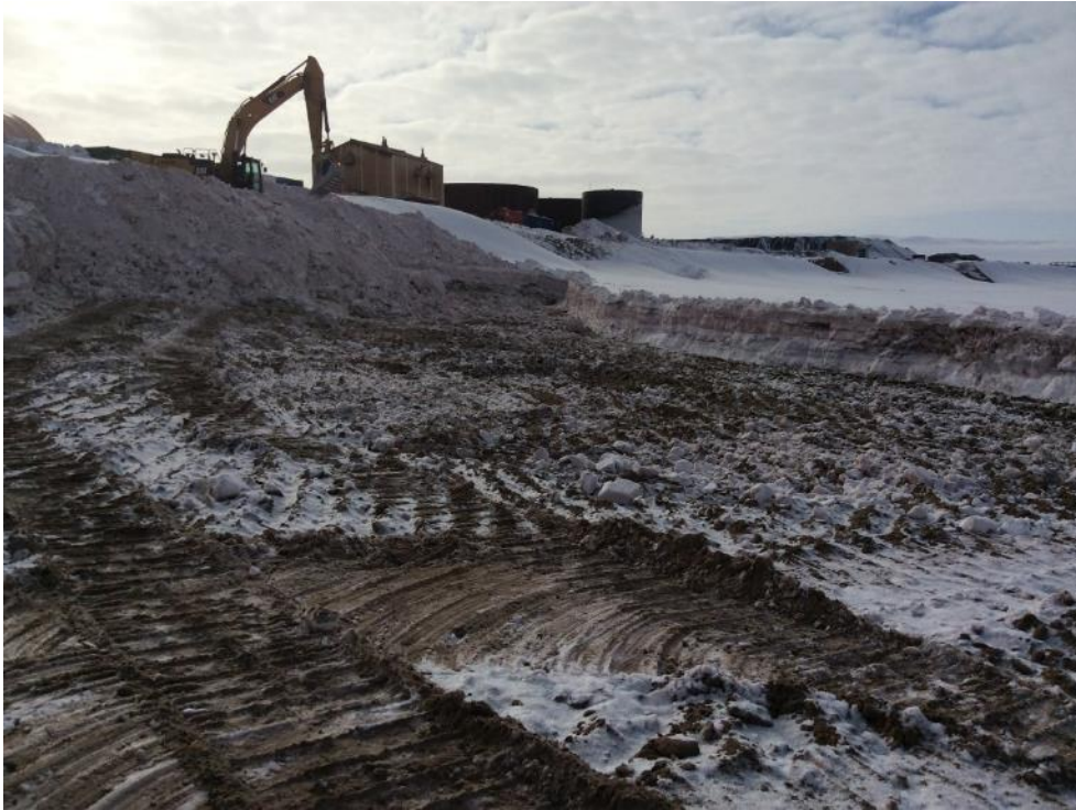
Photo 1 - Snow clearing for snow/sand rock containment berm to be built along the high-water mark shown at right side of the photo, 11 April 2019
