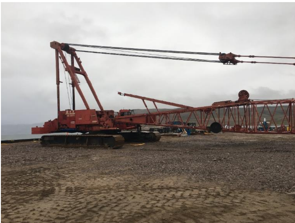
Photo 58 - Boom lowered on crane to be reconfigured, 29 July 2019
